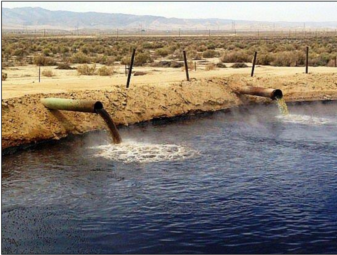
Figure 109: Unlined Wastewater Storage Pit 2 in Kern County, California.
