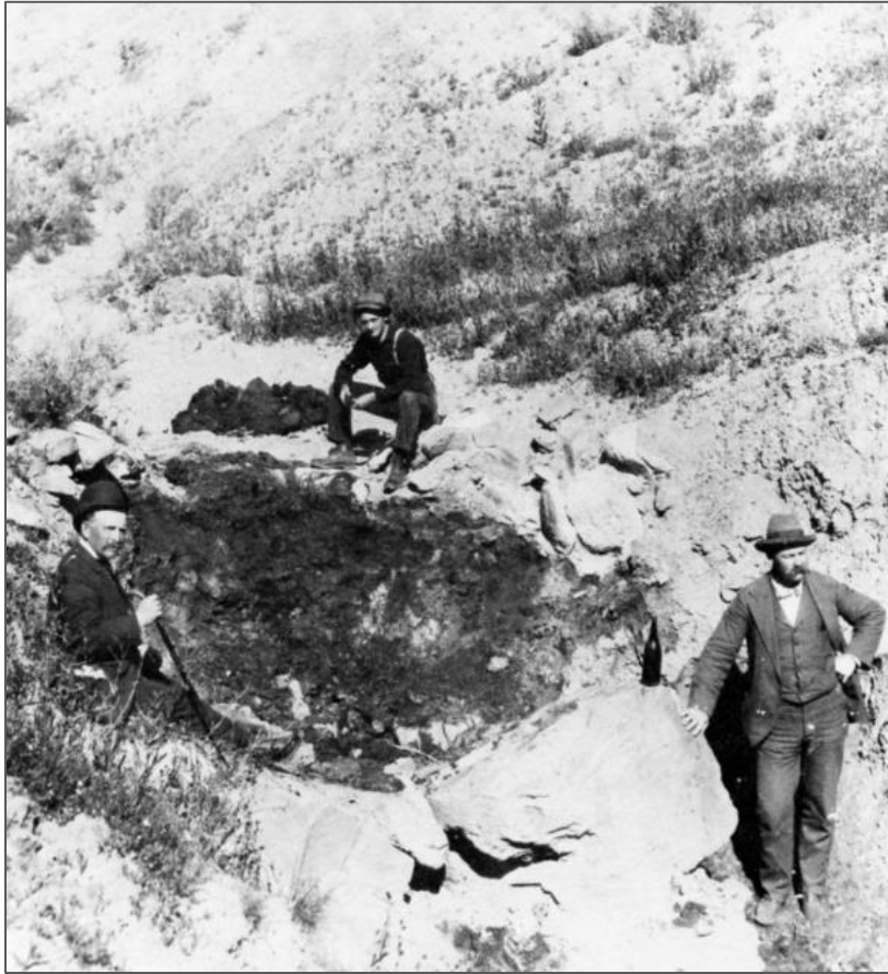
Figure 35: Pit and Tunnel Mining for Asphaltum in McKittrick, California.
