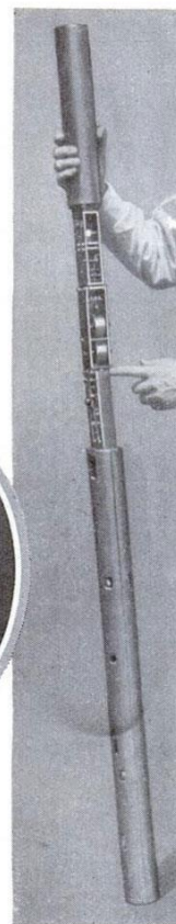
In circle, camera that makes records of film showing the inclination of well being dug. Right, whipstock that is set at bottom of well to deflect bit. Left, acid-etched bottle that shows slant of the well
