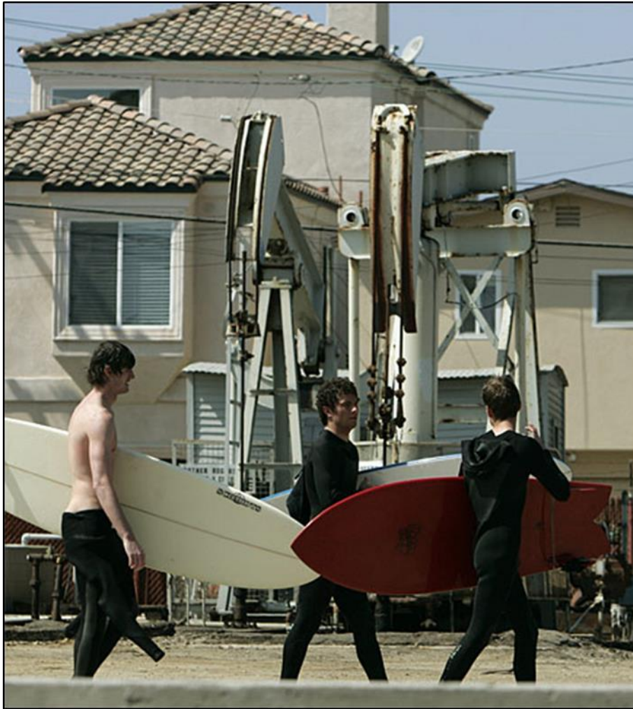
Figure 92: Pumpjacks Adjacent to Coastal Homes in Huntington Beach.
