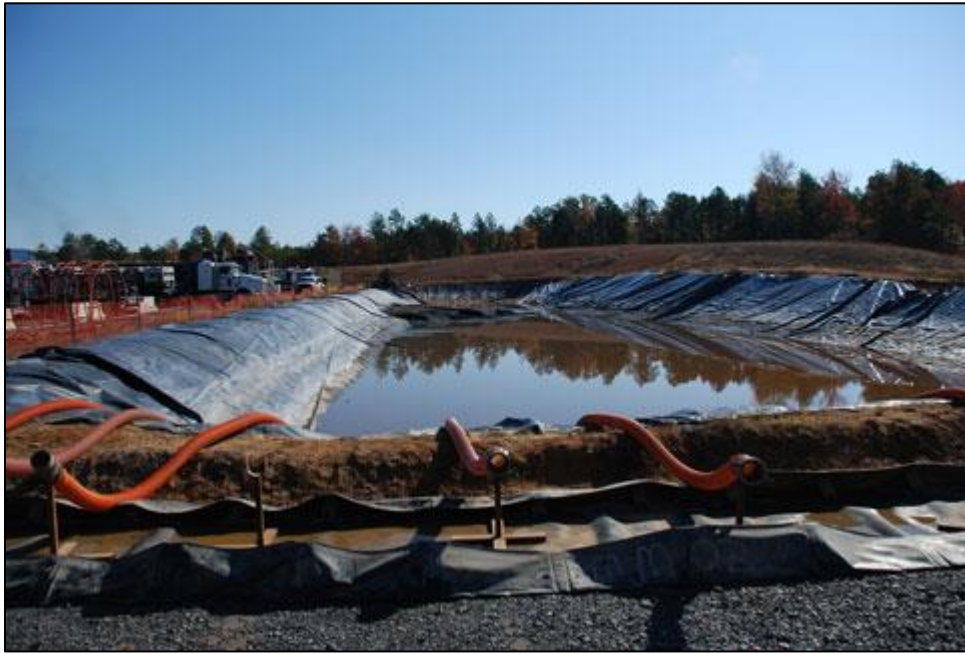
Figure 22: Lined Wastewater Storage Pit in Arkansas.
