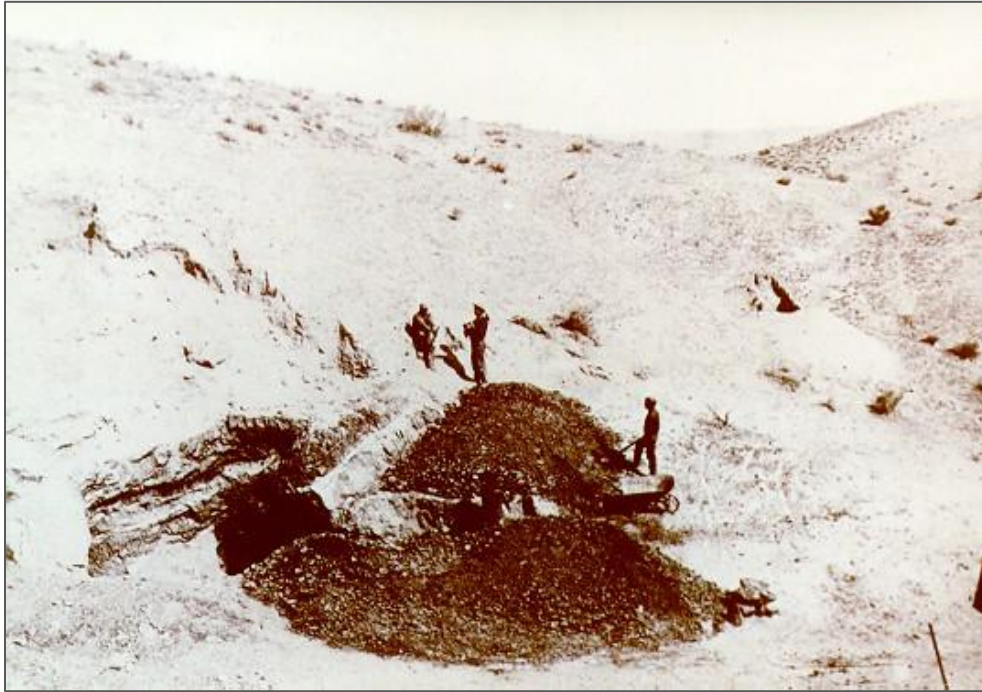
Figure 36: Asphaltum Excavation in McKittrick, California.
