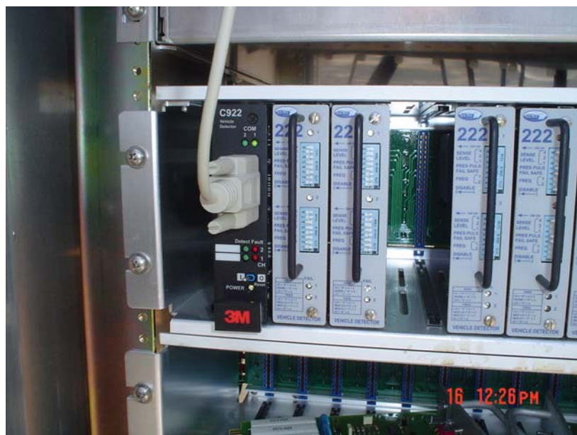
Figure 3.5. Laptop using RS232 serial interface with C922 3M Canoga Card
