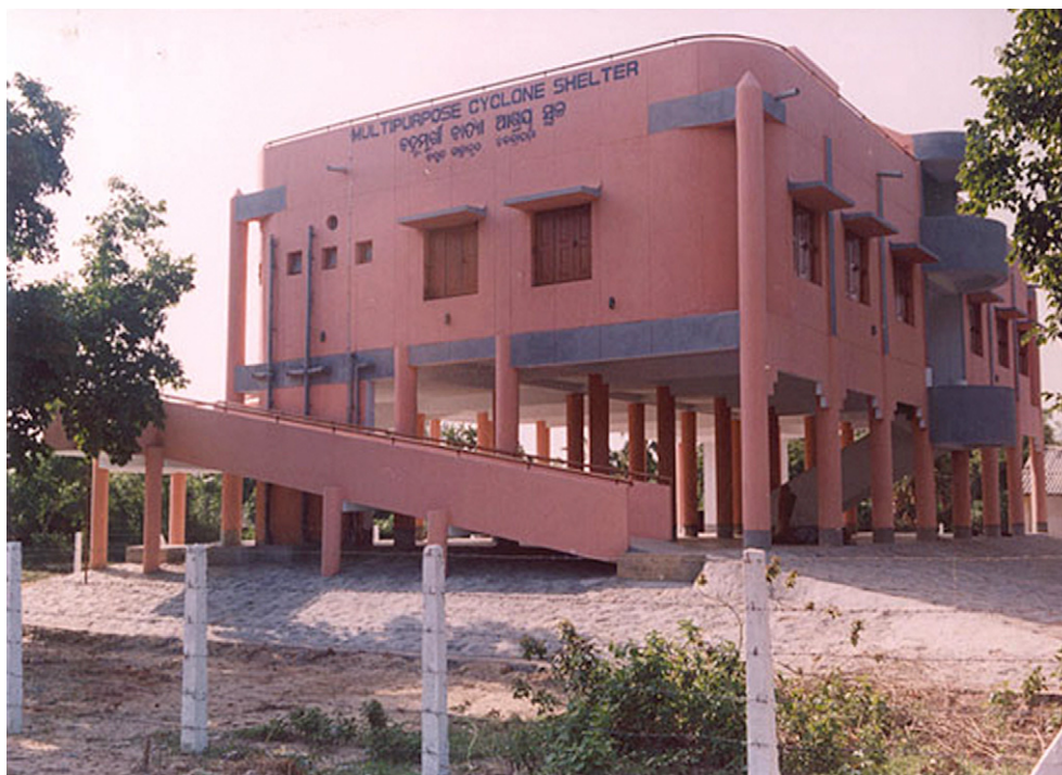
Fig. 3. Cyclone Shelter in Orissa Source: http://www.osdma.org/Photogallery.aspx?vchglinkid=GL025 , dt. 29.10.2009
