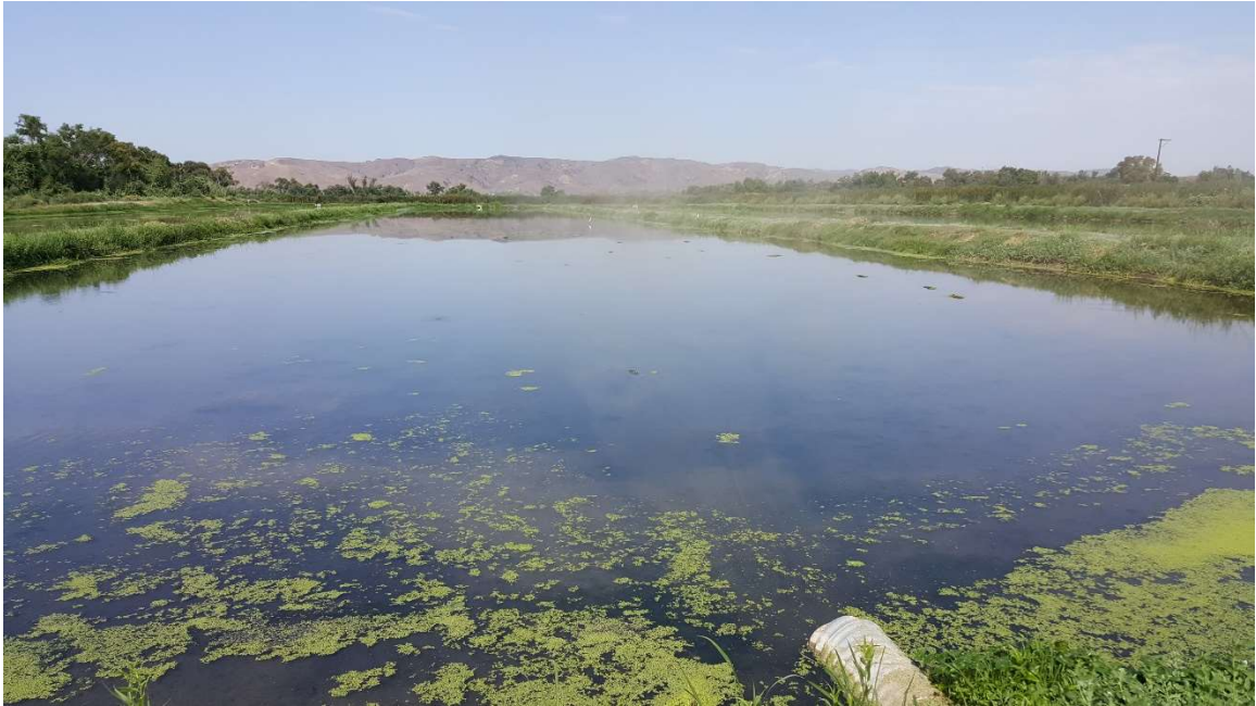
Figure 1.4: A unit process open water constructed wetland at the Prado Wetlands in Corona, California.
