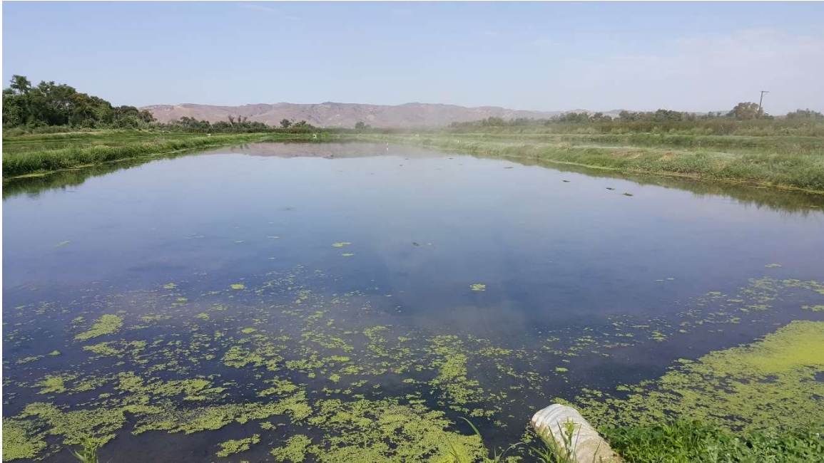
Figure 1.4: A unit process open water constructed wetland at the Prado Wetlands in Corona, California.
