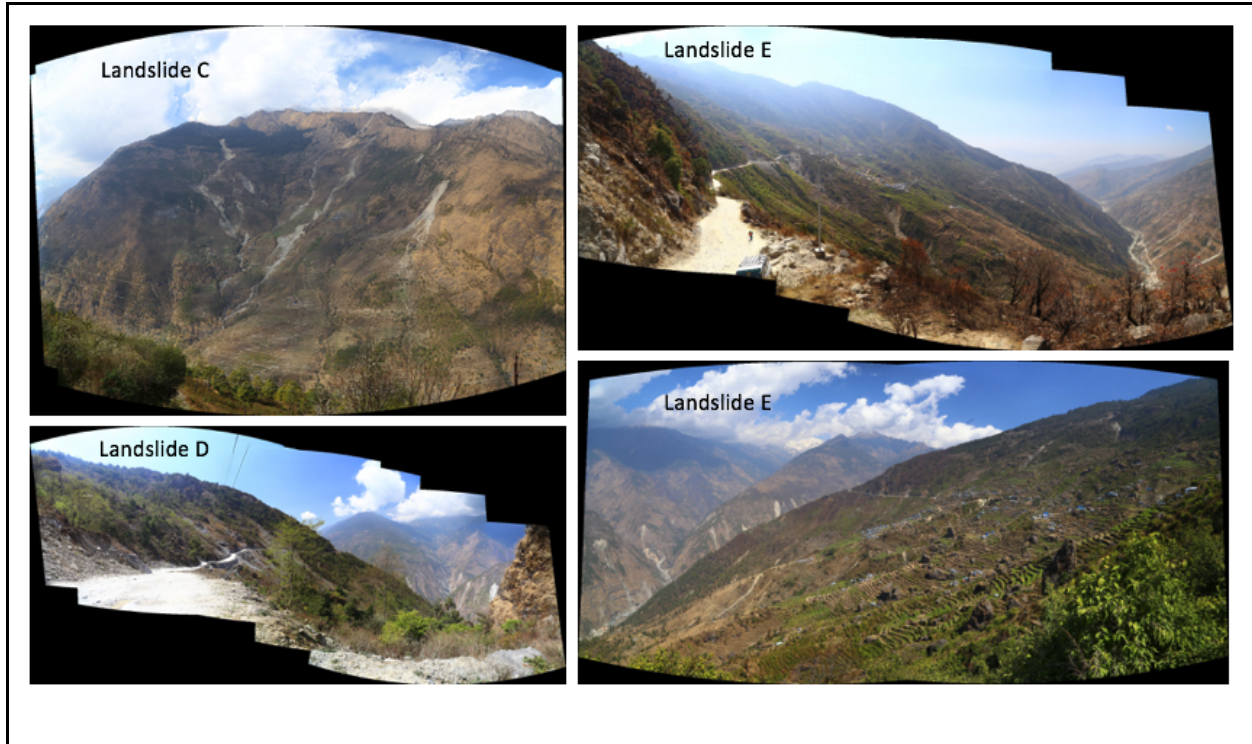
Figure S5: Field photos of landslides C, D, and E (see Figure 4 for location). Photos of landslide E are provided from two perspectives. The photos provide a ground based view of the landslides and show agriculture and ground surface deformation that is impacting the Trishuli highway (Photos courtesy of Jack G. Williams, Durham University).
