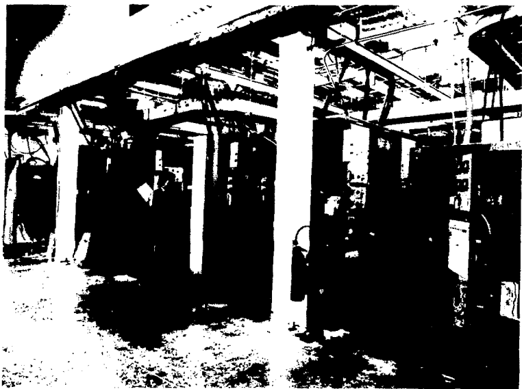
FIG. 12. Chopper power supplies located in Region 8 are rated either 300 or 840 kW and supply magnet power to all 20 magnet systems around the PEP ring. (CBB 801-904)
