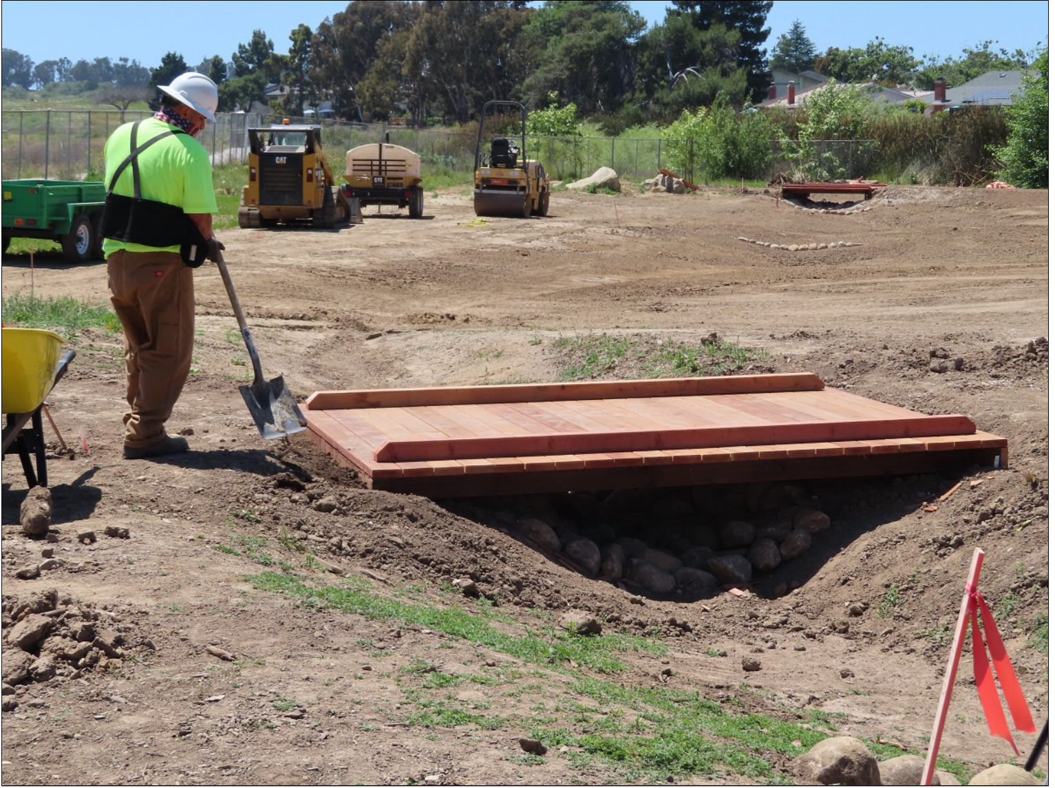
The Discovery Trail footbridges over the bioswales have recently been installed.
