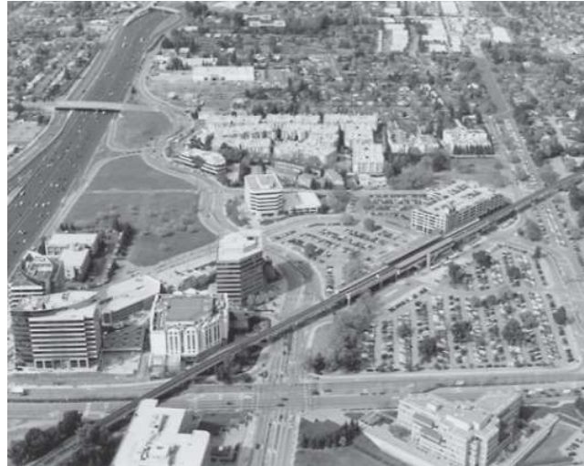
Figure 1: Pleasant Hill BART station and surroundings.
