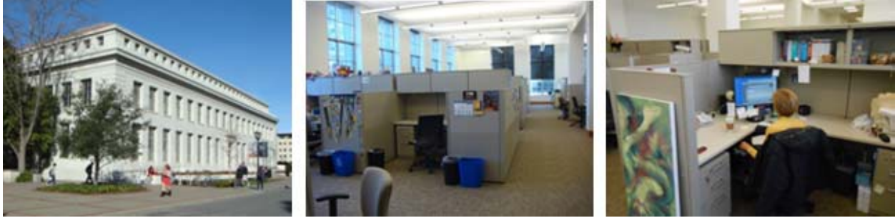
Figure 4.3-1 Photographs of Doe Annex Left – Exterior; Center – Interior View; Right – Typical Cubicle
