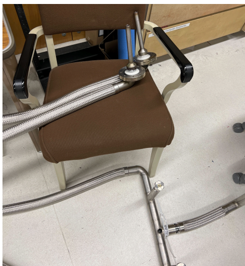
Figure 7a shows the transfer line with epoxy applied around the flange on both sides.
