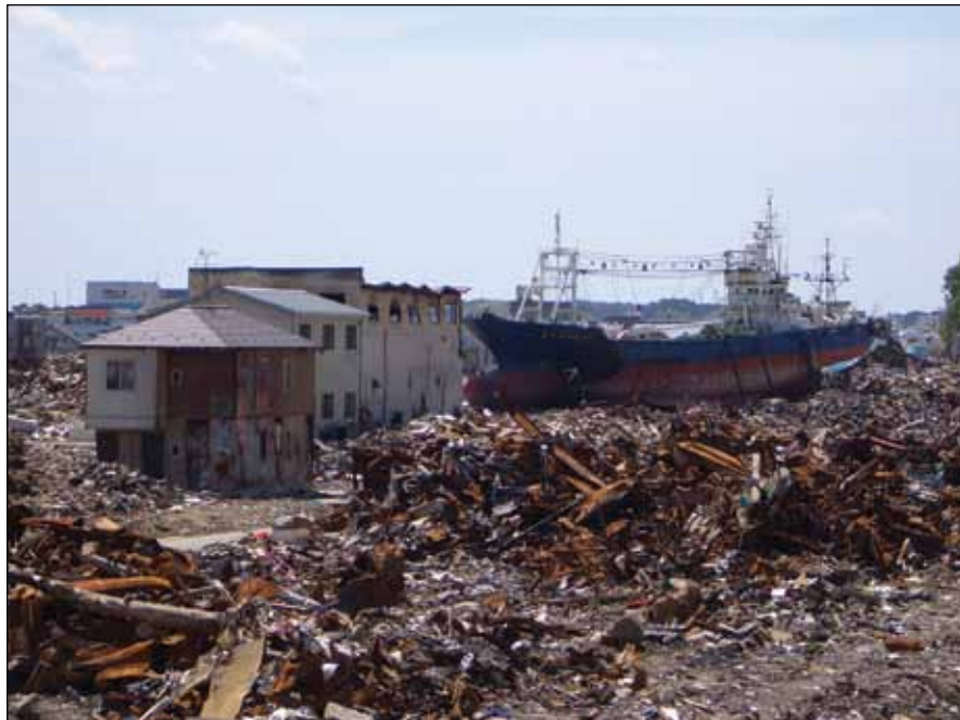
Plate 7: Roads were impassable due to damage and accumulation of a large amount of debris (photo taken in Kesenuma).
