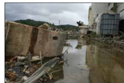
Plate 8: (A – top) Flooding in an area near the coastline due to land subsidence (photo taken in Minami-sanriku), (B – bottom) and a road underwater (photo taken in Ishinomaki).
