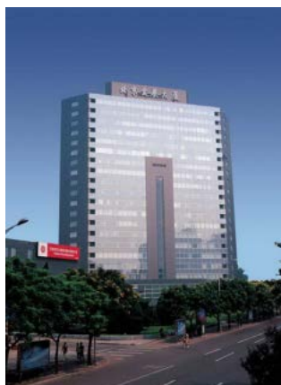
Fig 2. A Photo of Building B.
