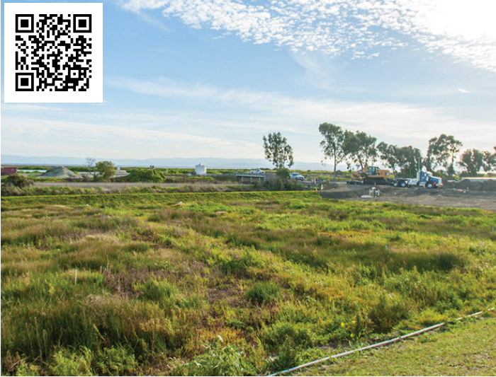
Figure 1: Horizontal levee in Oro Loma created as part of the NSF's ReNUWIt project is an example of nature-based water treatment. Scan the QR code for a video of the site's construction and an overview of the coastal protection offered by the levee.
