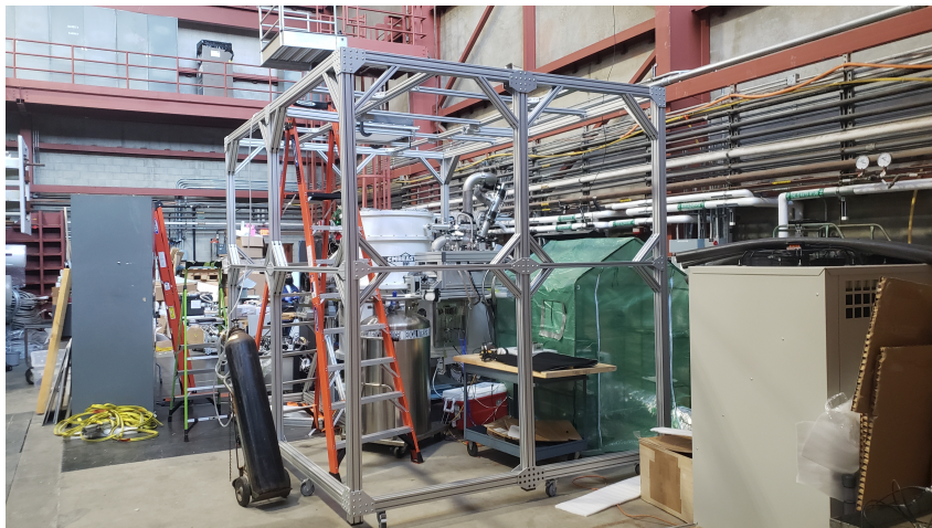
Figure 5.4. Photo of test equipment mounting frame, built out of T-slot aluminum.
