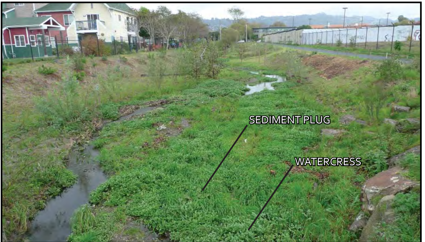
FIGURE 13. PHOTOGRAPH OF PHASE 3 NEAR RS 14+00
