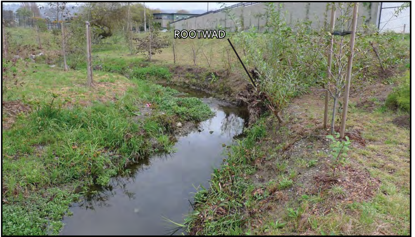
FIGURE 14. PHOTOGRAPH OF PHASE 3 NEAR RS 16+40.
