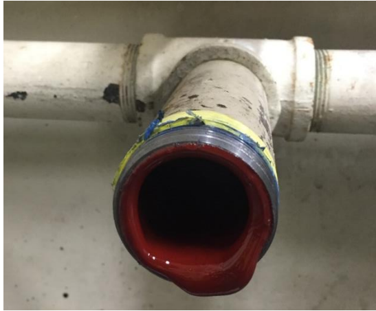
Figure 16: Pipe fitting coated with the copper epoxy
