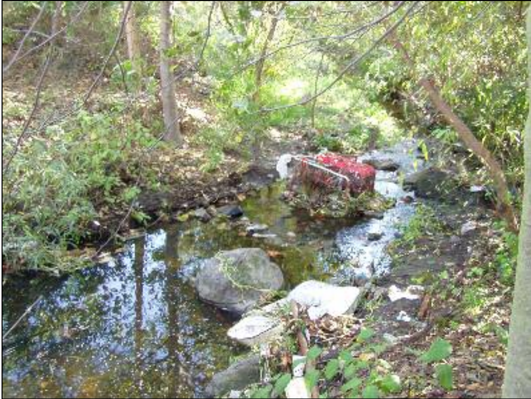
Figure 15: 50 ft from upstream culvert (looking downstream)
