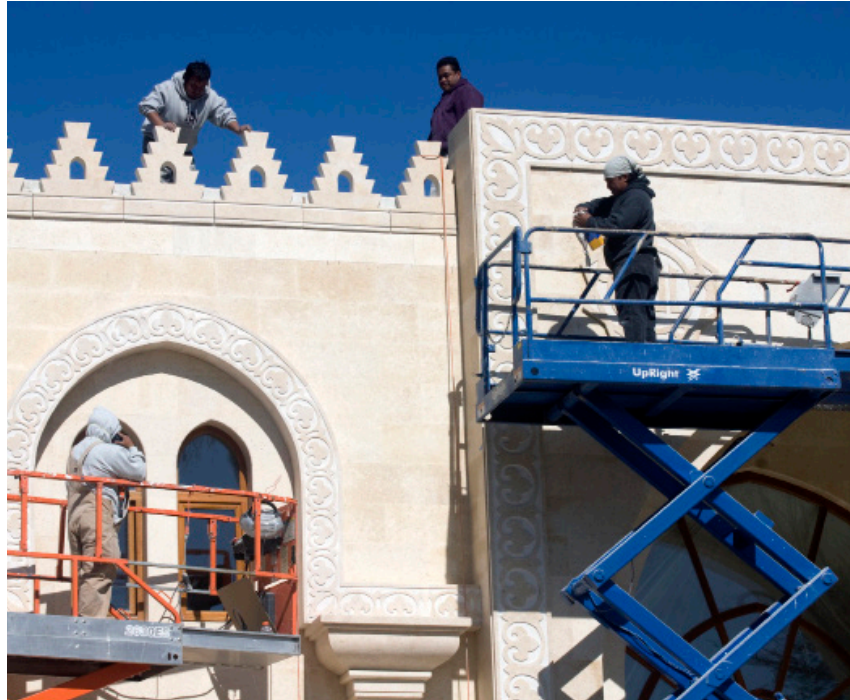
Figure 14: The application of architectural details from the Fatimid Masjid. Source: Courtesy of Najam Alanwar.
