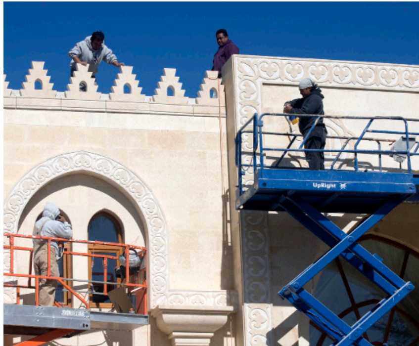
Figure 14: The application of architectural details from the Fatimid Masajid. Source: Courtesy of Najam Alanwar.
