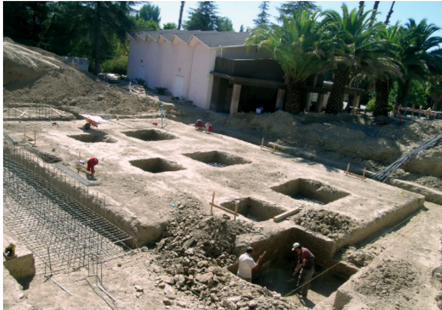
Figure 32: Construction phases for the masjid. Source: Courtesy of Najam Alanwar.
