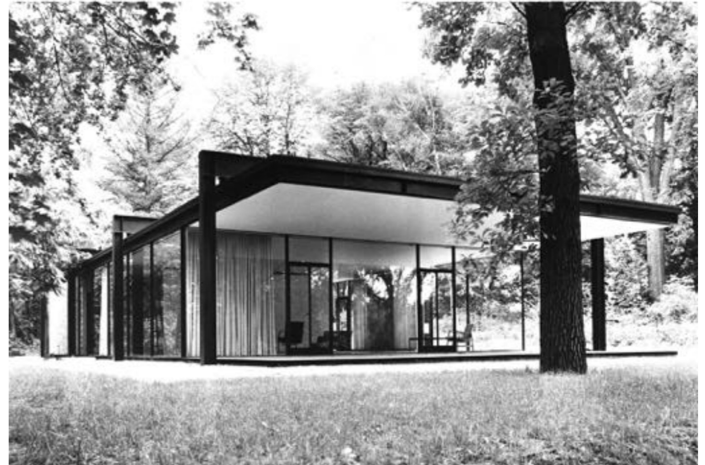
Figure 1: South Elevation, Graham Resource Center, Illinois Institute of Technology. (Source: J. C. Brownson, Master's thesis, IIT, 1954.)
