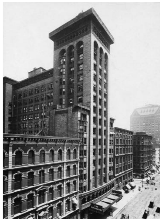
Figure 2a (from top): Adler & Sullivan, Auditorium building, Chicago 1889; Adler & Sullivan, Schiller building, Chicago 1892. (Source: Ryerson and Burnham Archives, the Art Institute of Chicago.)
