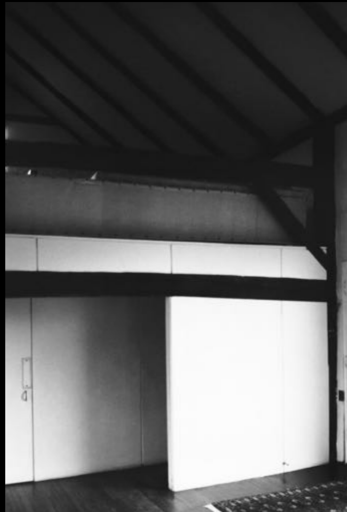
Figure 5: The Living Barn, post and beam structure, 1975. (Source: Ludwig Glaeser, photographer. Canadian Centre for Architecture, with kind permission by Nicolas Köhler.)
