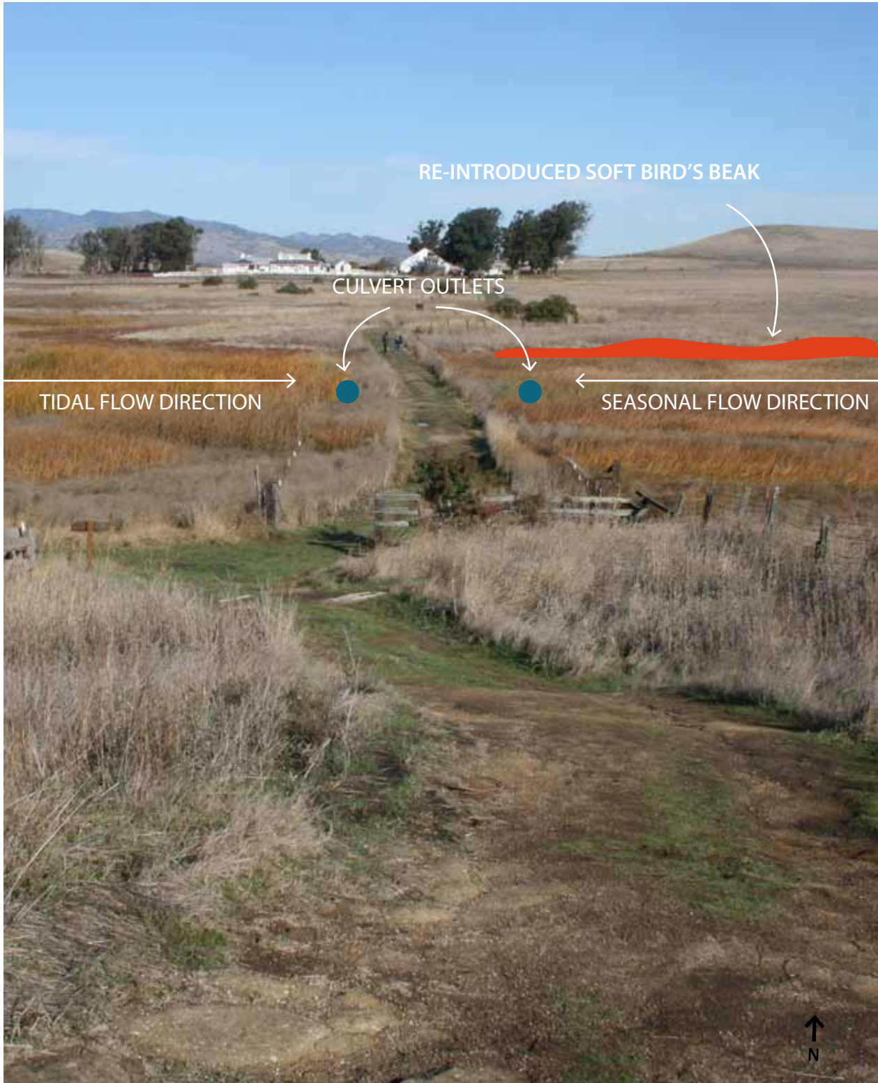
SITE PHOTO OF LOWER SPRING BRANCH CREEK LEVEE
