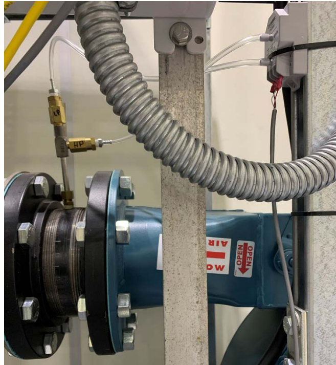
Figure 7.6 – Differential Pressure Transducer with Pitot Tube.
