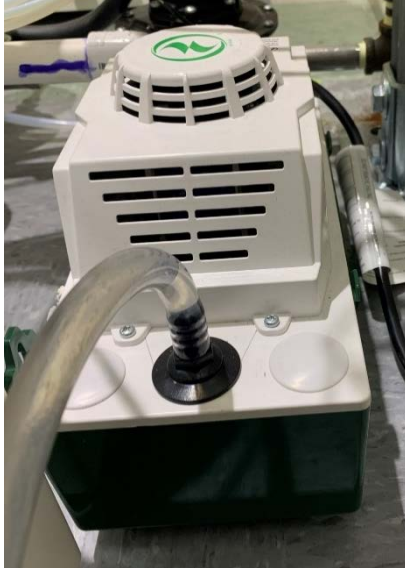
Figure 6.14 – BlueGEN Drainage Sump Pump.
