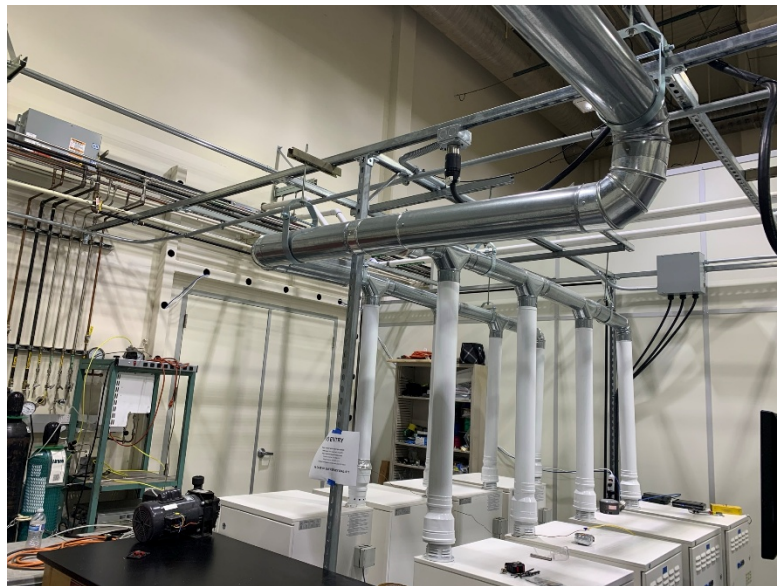
Figure 6.10 – BlueGEN Exhaust Manifold.
