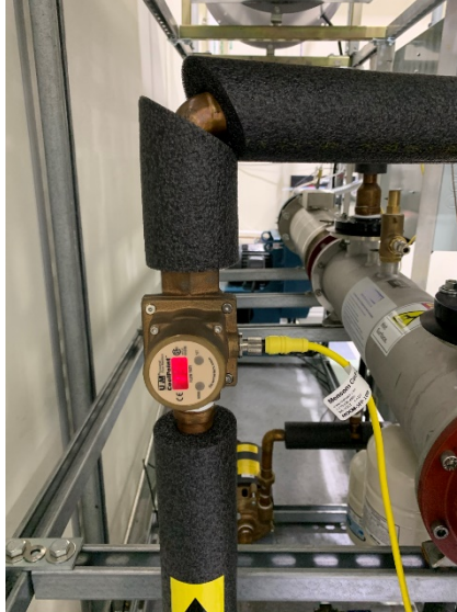
Figure 7.5 – Hot Water Flow Meter.
