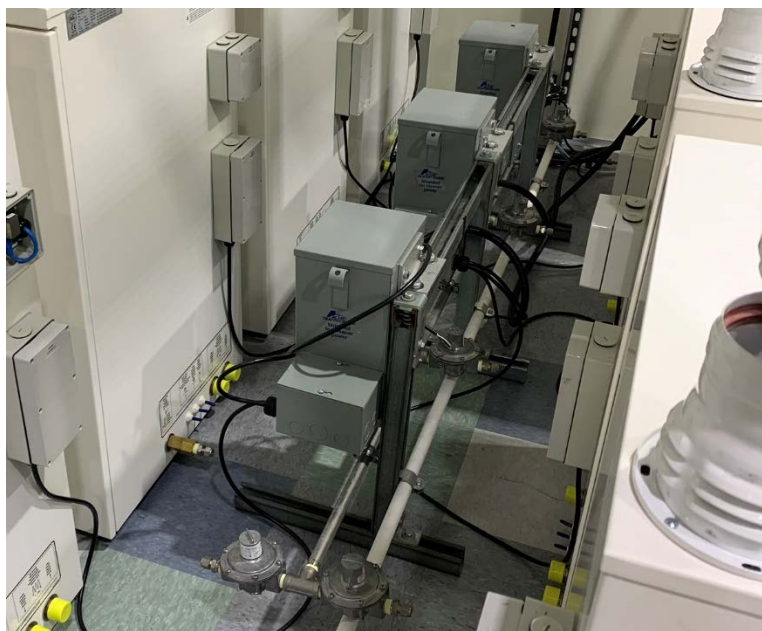
Figure 6.9 – BlueGEN Systems NG Connection Manifold.
