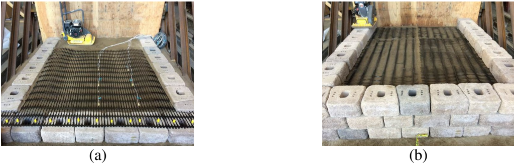
Figure 4. Construction of GRS bridge abutment: (a) longitudinal reinforcement; (b) transverse reinforcement.
