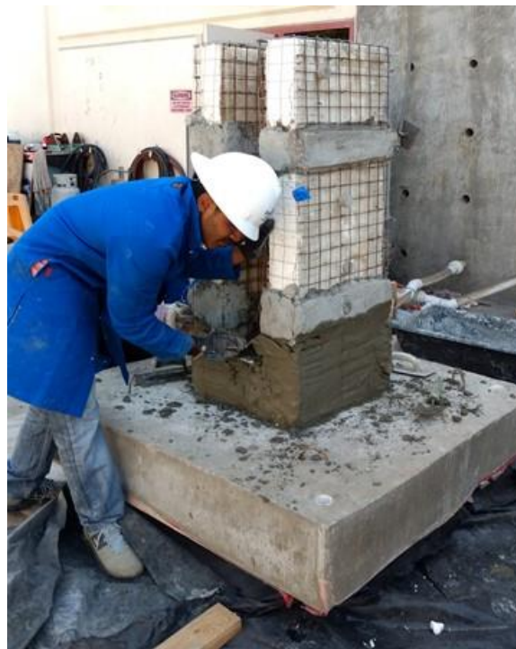
Figure (3.10): Hand-applied Mortar on I-Section Column
