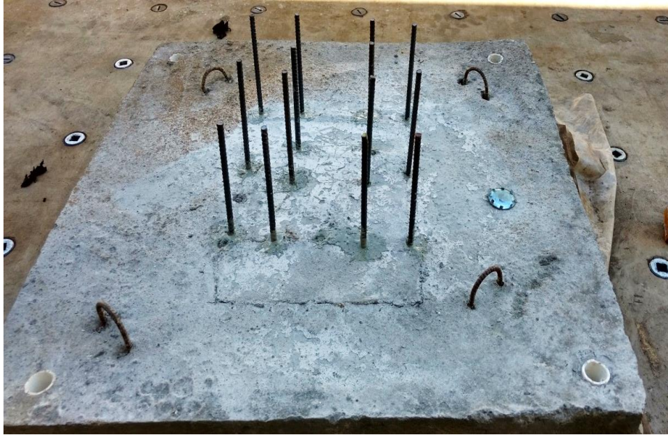
Figure (3.8): #4 Rebars Installed to Foundation Using High-Strength Epoxy
