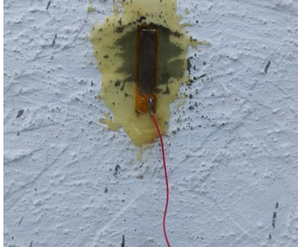
Figure (3.19): Strain Gauge Installed on Mortar Surface of Columns
