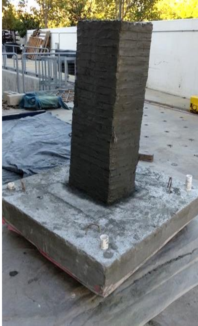
Figure (3.13): Hand-applied mortar on Asymmetric C-Section Column
