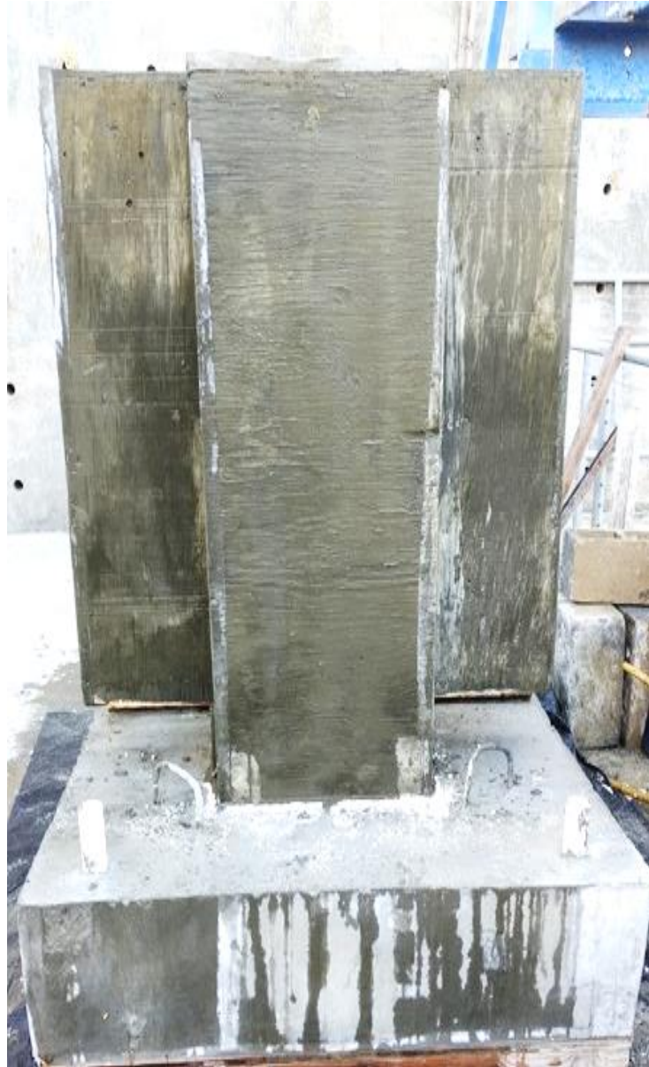
Figure (3.12): Hand-applied mortar on symmetric I-Section Column
