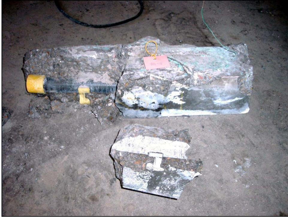
Figure 21. Extraction of dowels for visual inspection.
