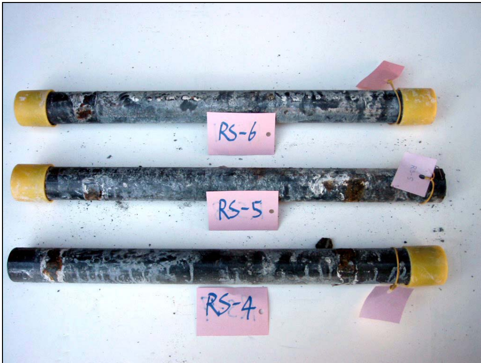
Figure 22. Corrosion along the carbon steel bars.
