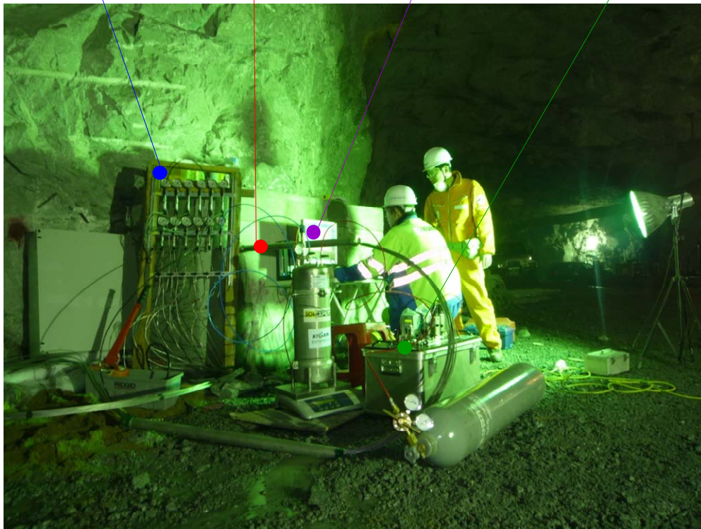
Figure 6. (a) Schematic drawing and (b) installation at the cavern of the pilot plant for CAES of in-situ permeability measurement system for concrete lining and surrounding rock mass.
