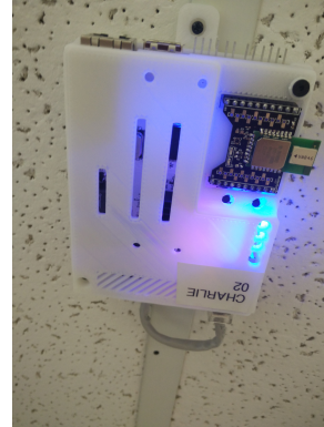
Figure 7.6: A version 2 NTB device mounted to a lab ceiling and powered via ethernet (PoE).
