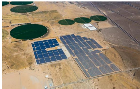
Figure 28: Sunray Energy Project 2 and 3 replaced SEG I & II (Photo: Clēnera. 2017)
