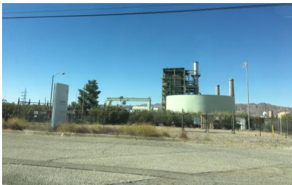
Figure 27: Coolwater Generating Station (Photo: Author, 2020)
