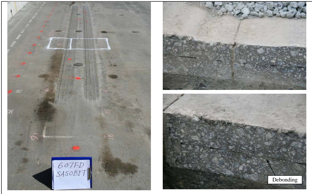
Figure 5.17: 607FD: Test pit photographs.
