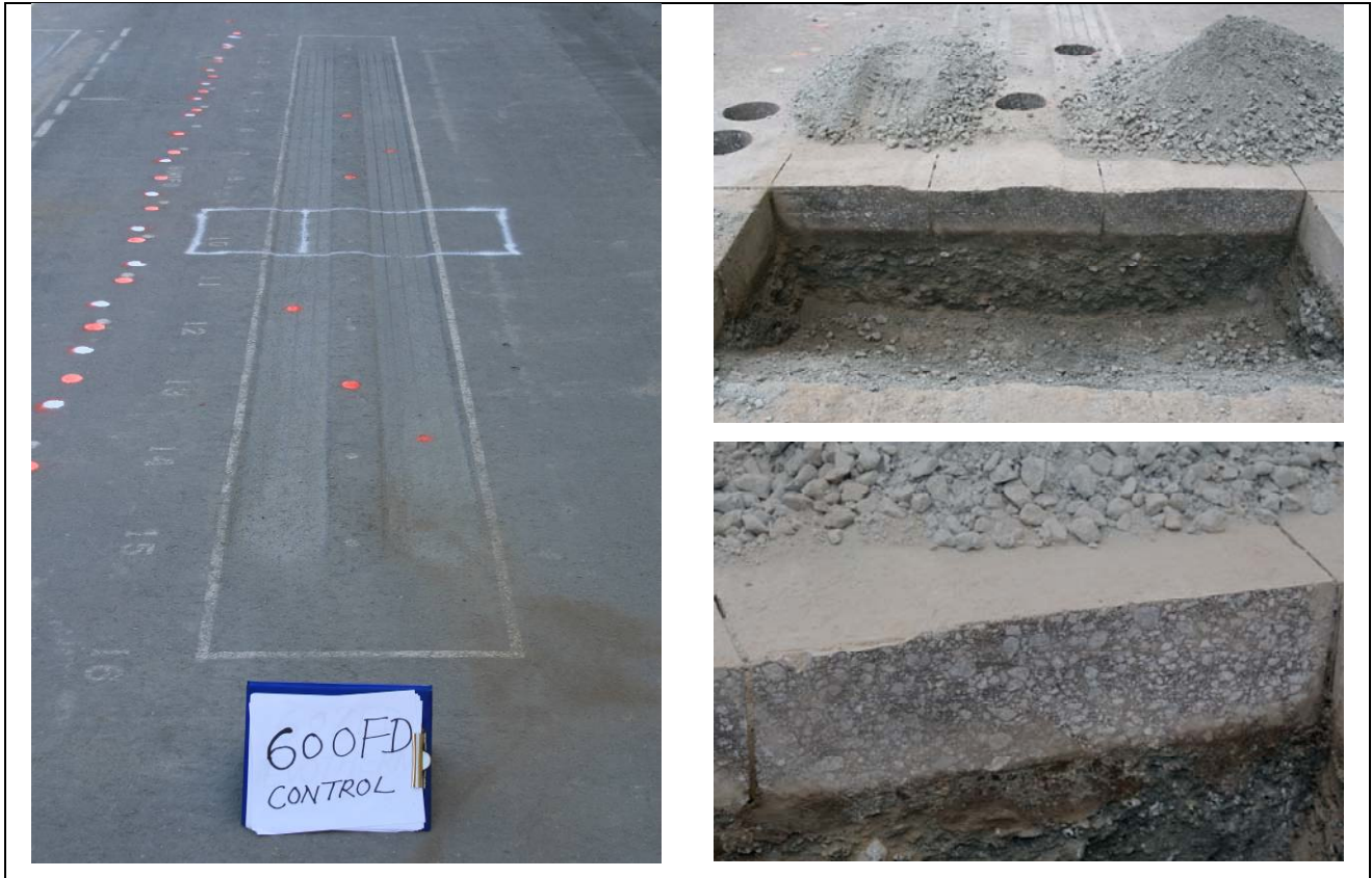
Figure 5.10: 600FD: Test pit photographs.
