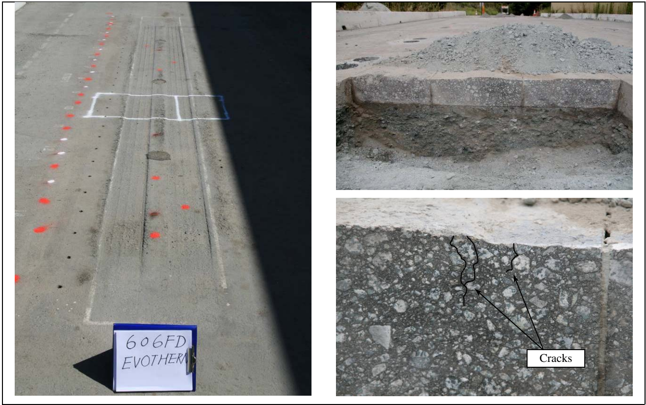
Figure 5.16: 606FD: Test pit photographs.
