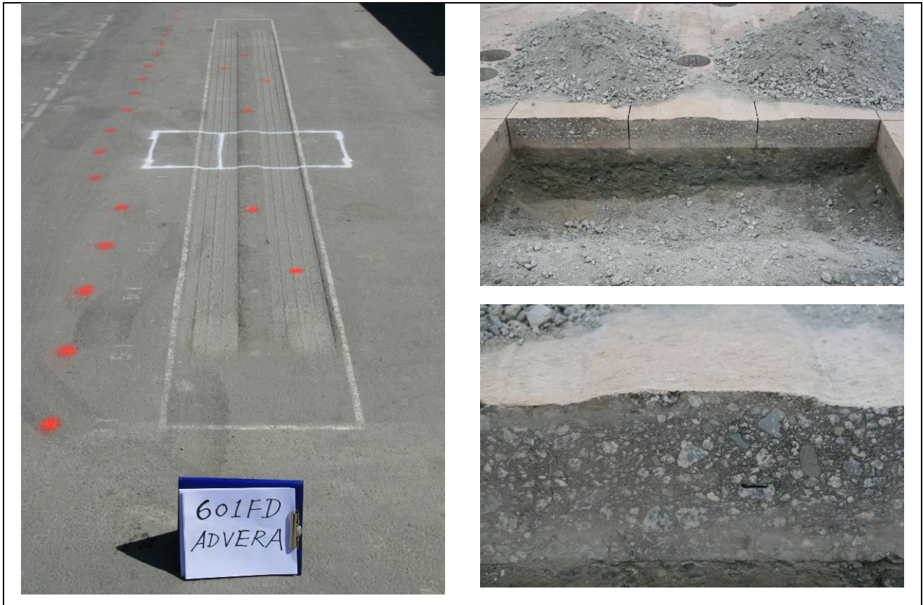
Figure 5.11: 601FD: Test pit photographs.
