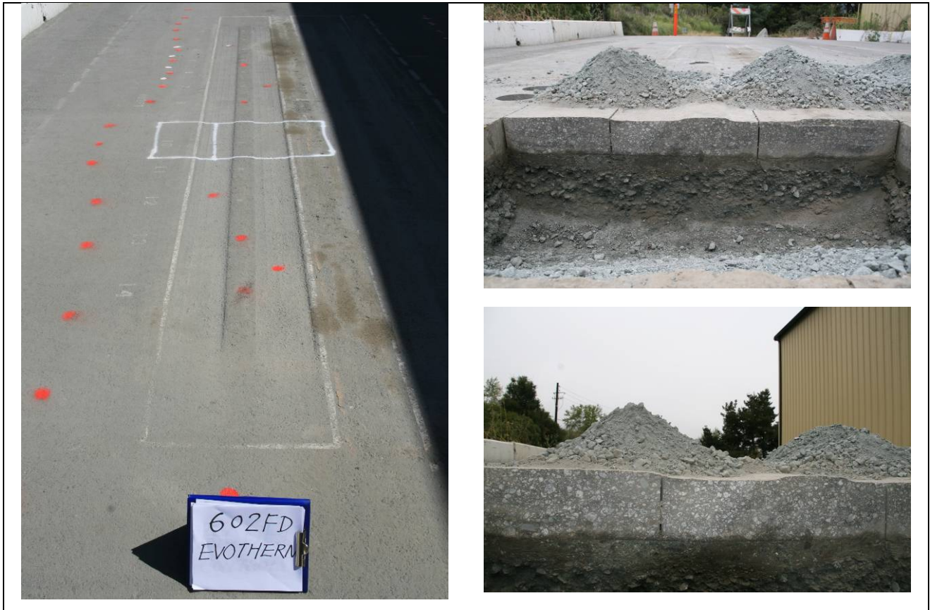
Figure 5.12: 602FD: Test pit photographs.
