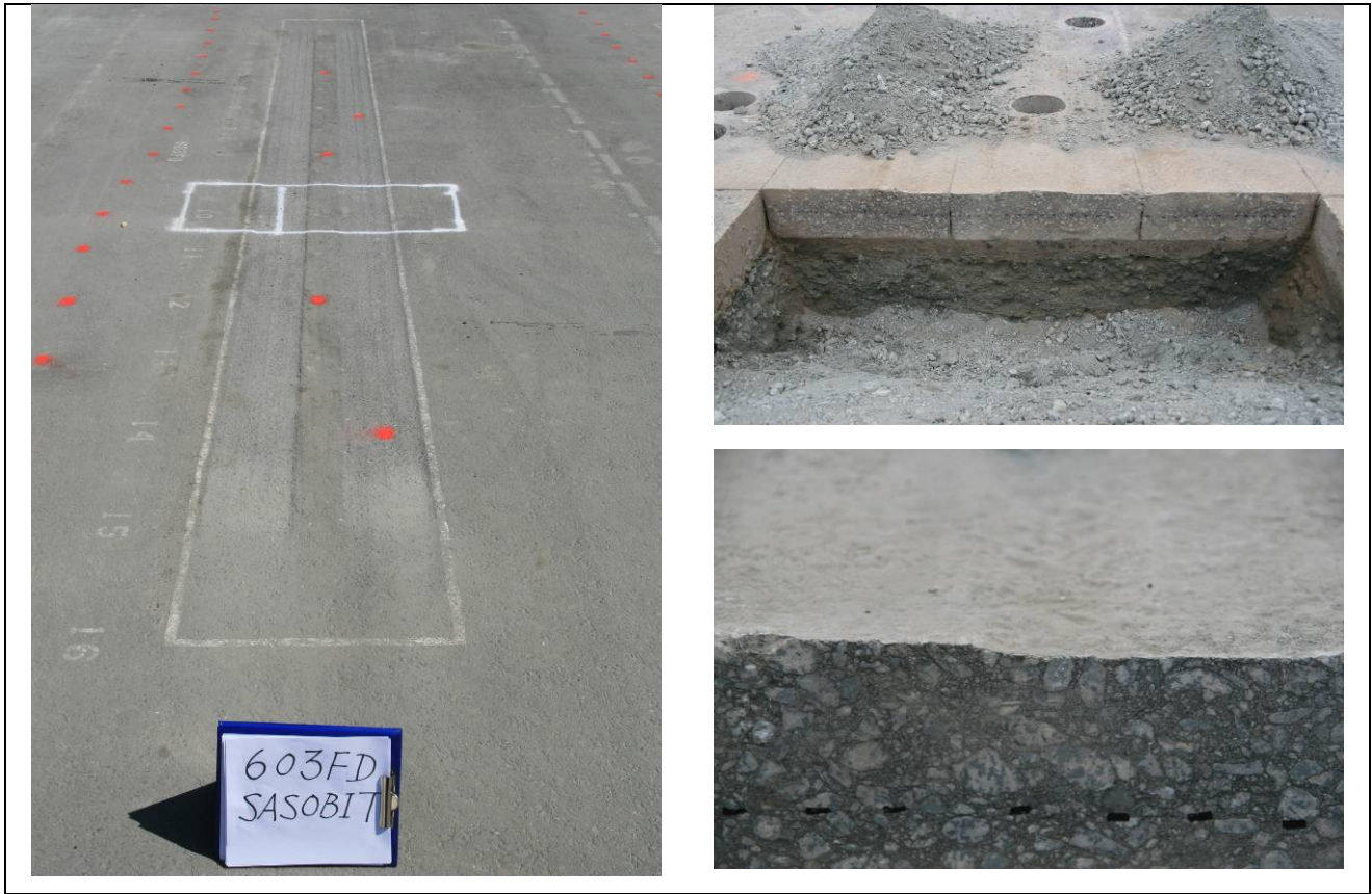
Figure 5.13: 603FD: Test pit photographs.
