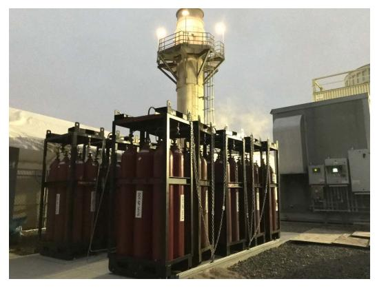
*Figure 88. Siting of the six-pack hydrogen cylinders at the UCI Central Plant on concrete pad space.*
