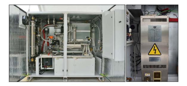
*Figure 4. C10 electrolyzer system. Fluids cabinet containing mechanical systems and cell stack on the left, electrical cabinet containing the power electronics on the right.*
