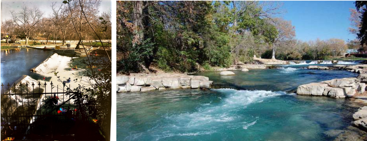
Figure 7 (left): Photograph of Rio Vista Dam before renovations in 2006.
