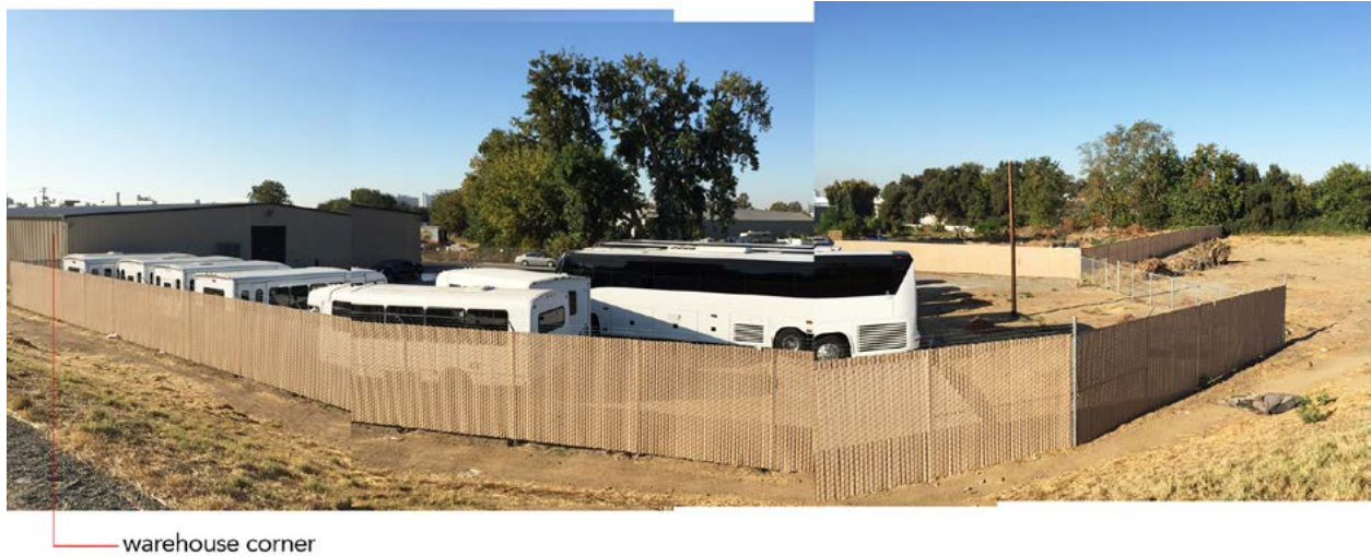
Figure 6.3 Property looking south from the top of the levee, October 2018
