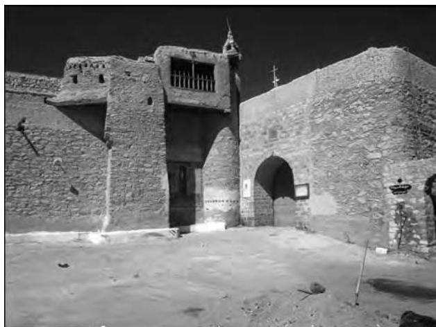
Figure 23.4. The outer walls of Saint Paul's Monastery. The fatuli is in the covered room with the large balcony above the icon of Saint Paul. Photograph by Patrick Godeau, ARCE 97-1126-19.
