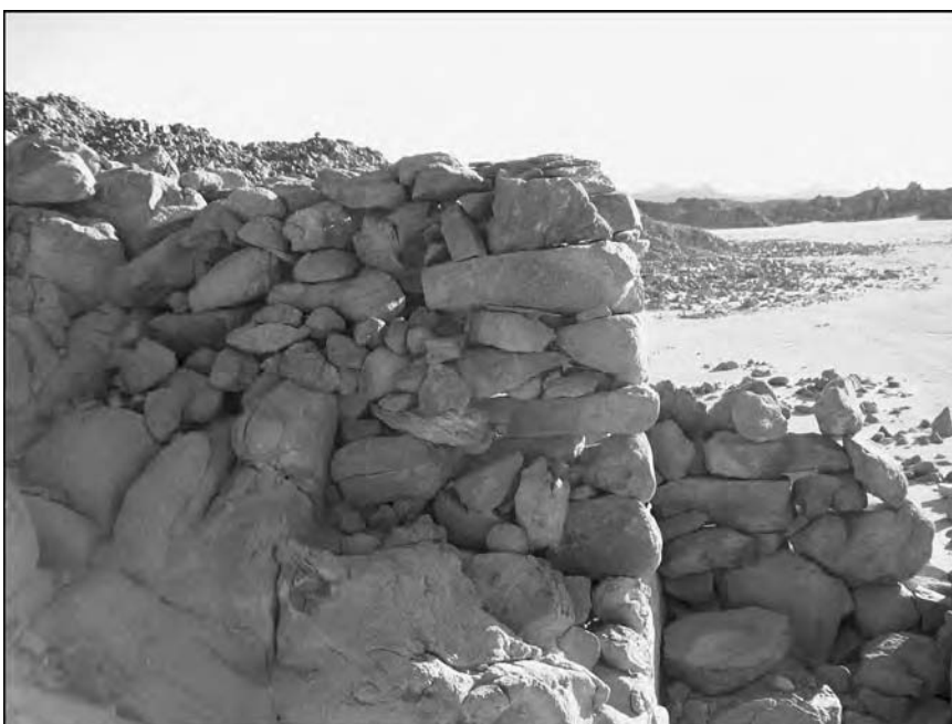
Figure 15.8. The building identified as a shrine near the ancient gold mining settlement in Wadi Bakariya, Central Eastern Desert, Egypt.
