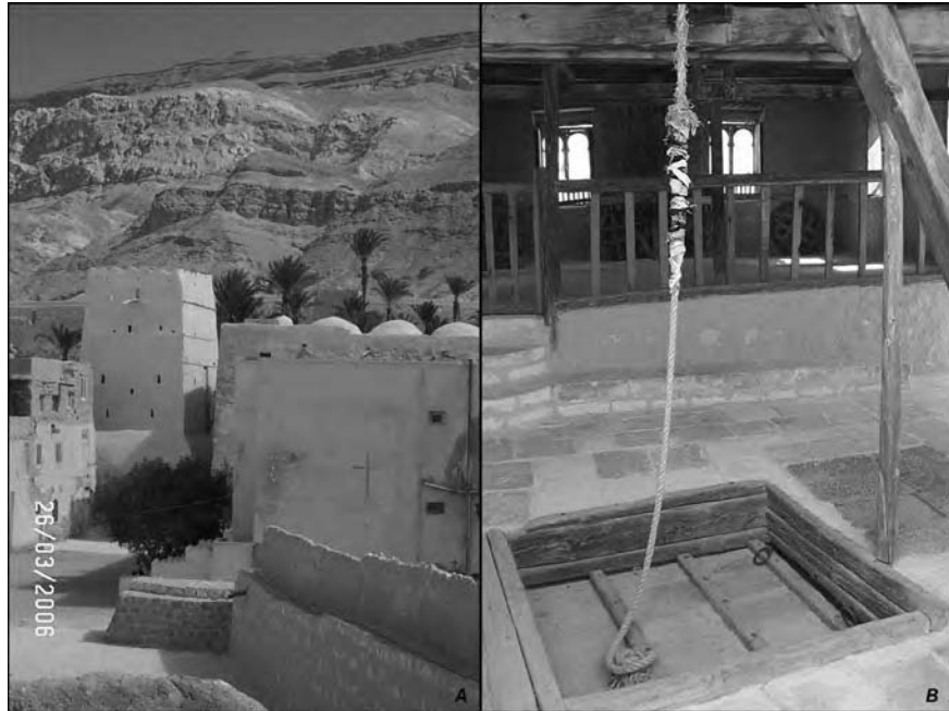
Figure 22.7. a: Keep and monastic cells at Saint Anthony's Monastery. b: Hoist and pulley forming the former entrance to the monastery.
