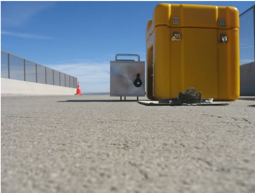
Figure 4.142: Surface and joint on Section QP-163.1.
