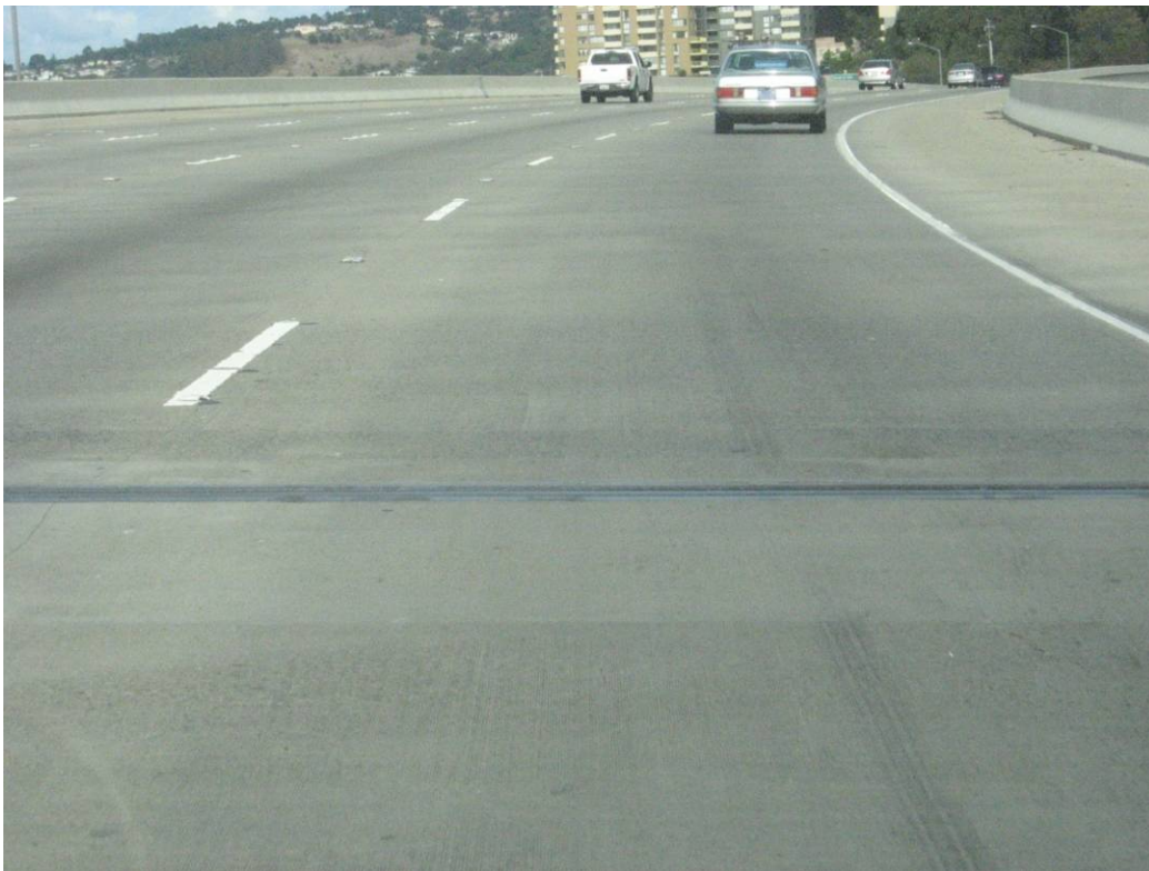
Figure 4.20: Surface and joint on Section QP-120.1.
