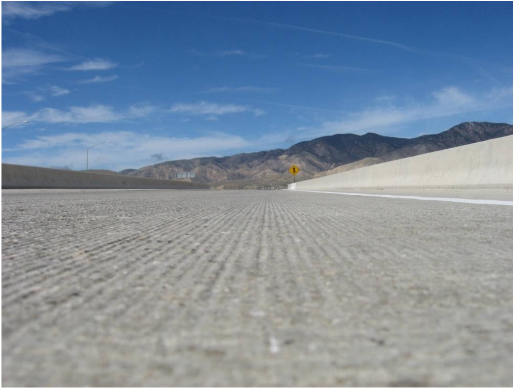
Figure 4.149: Surface texture on Section QP-164.1.
