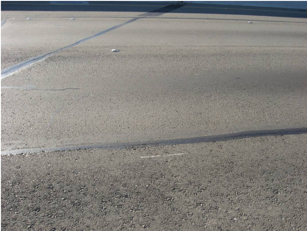
Figure 4.112: Surface and joint on Section QP-150.1.
