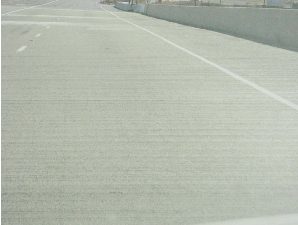
Figure 4.42: OBSI Surface and diamond-ground segments near joints on Section QP-124.1.
