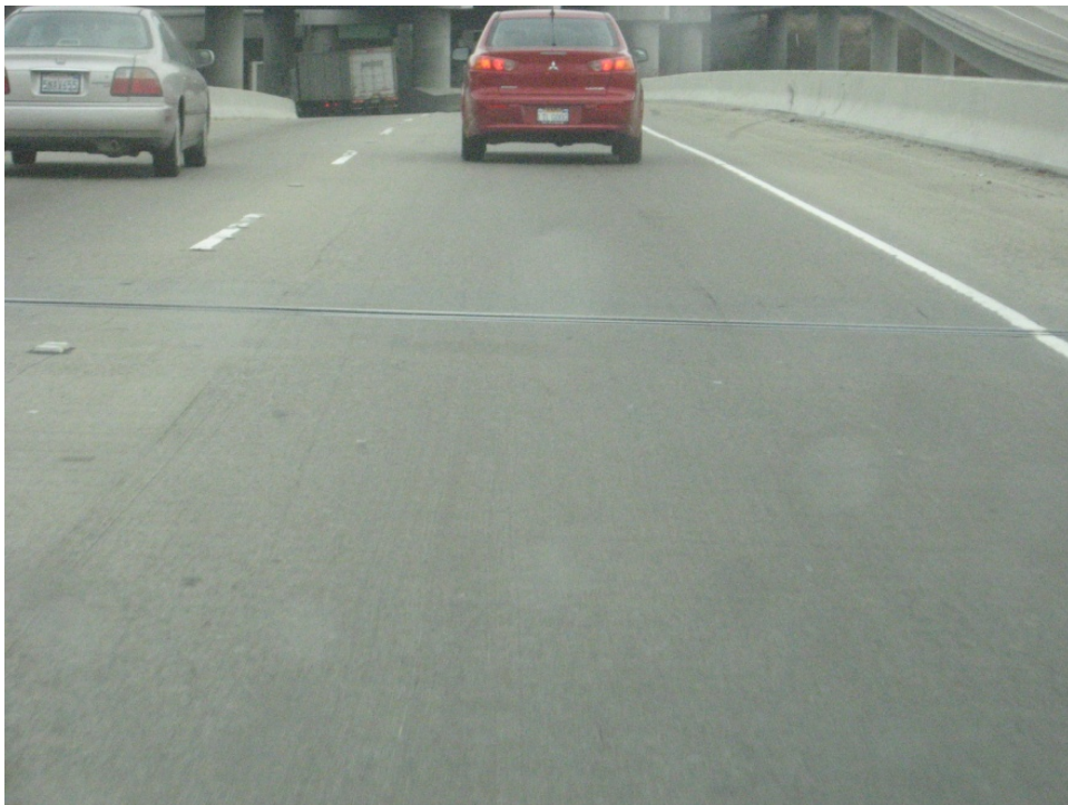
Figure 4.2: Surface and joint on Section QP-118.1.
