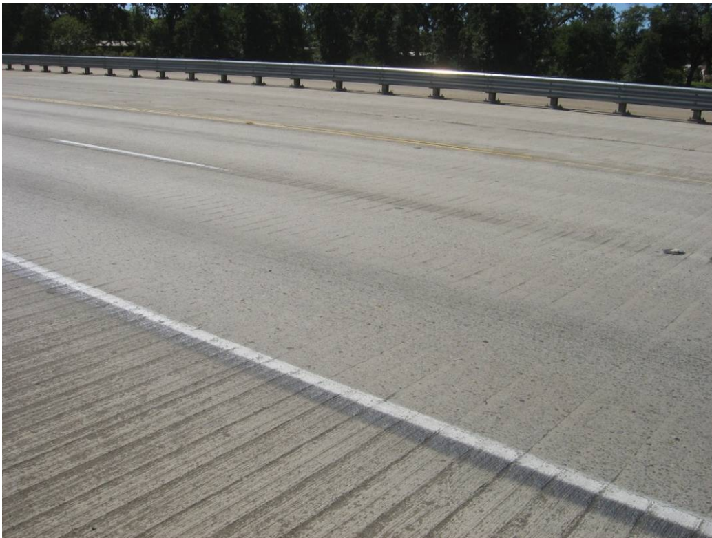
Figure 4.75: Texture difference in the wheelpath and the rest of bridge deck on Section QP-141.1.
