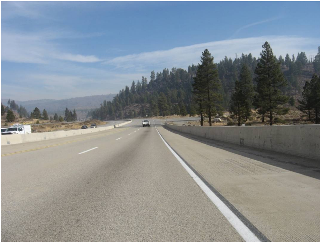
Figure 4.84: Surface of Section QP-143.1.
