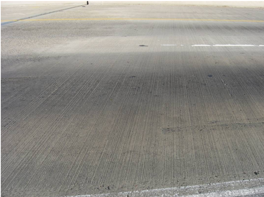
Figure 4.128: Surface and joint on Section QP-152.1.
