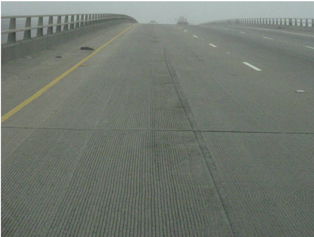
Figure 4.119: Surface and typical joint on Section QP-151.1.
