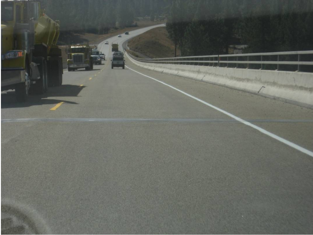
Figure 4.99: Surface and joint on Section QP-145.1.
