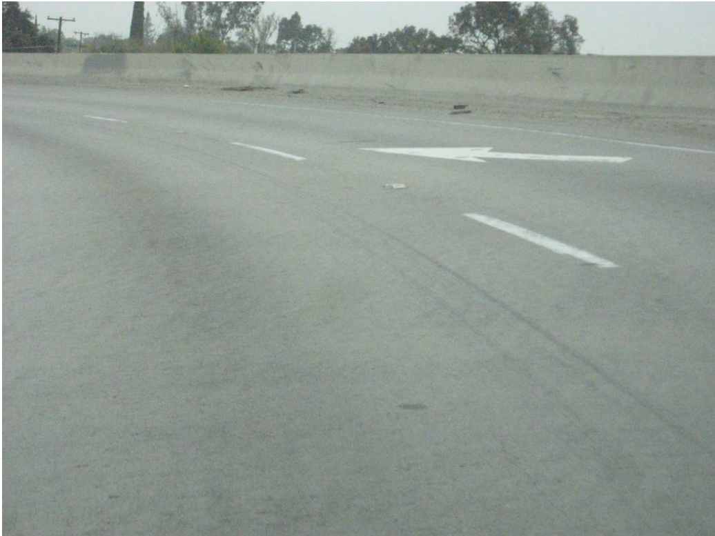
Figure 4.107: Surface of Section QP-149.1.
