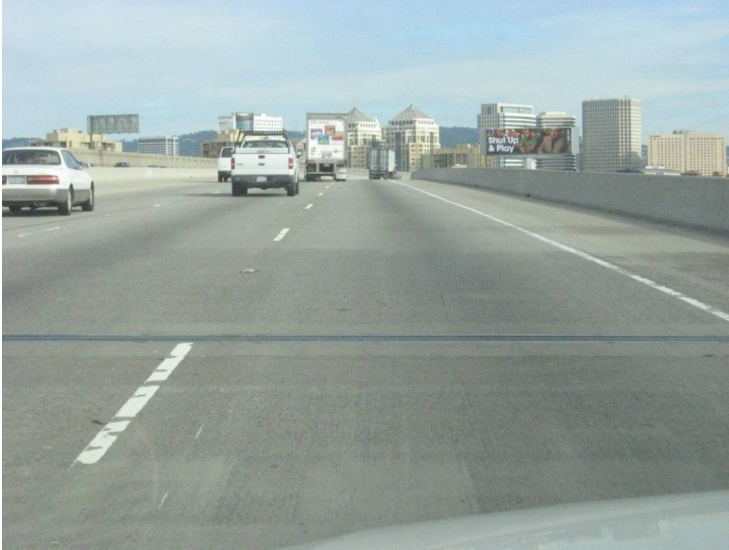
Figure 4.35: Surface and joint on Section QP-122.1.
