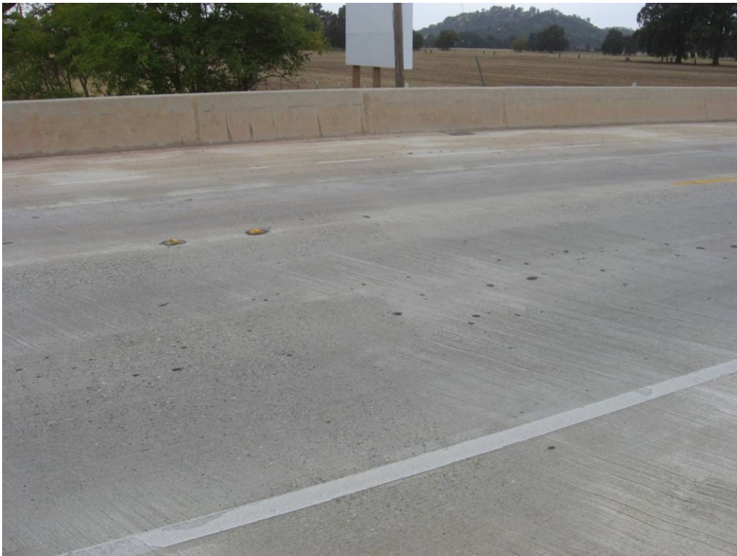
Figure 4.68: Surface and joint on Section QP-140.1.
