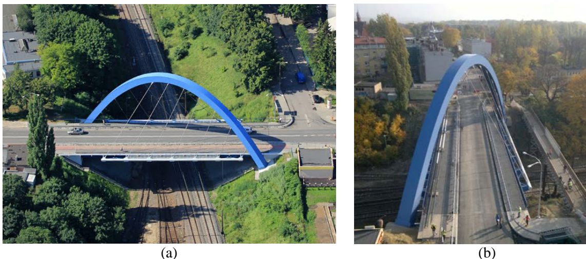
Figure 12: Wiadukt in Tczew, Poland: (a) side view [11], (b) end view [12].
