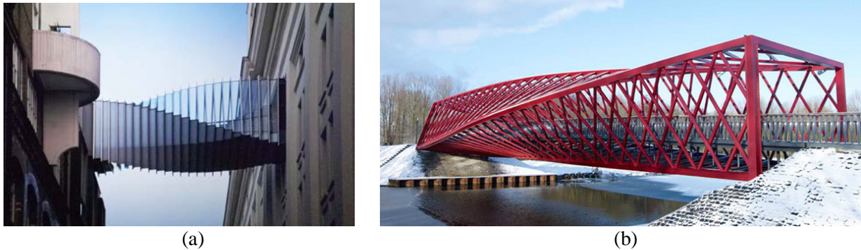
Figure 18: Twisted bridges: (a) Floral Street Bridge, Covent Garden, London [16], (b) bridge from Holy-Zuid district to the Broekpolder over Vlaardingse Vaart in The Netherlands [17].
