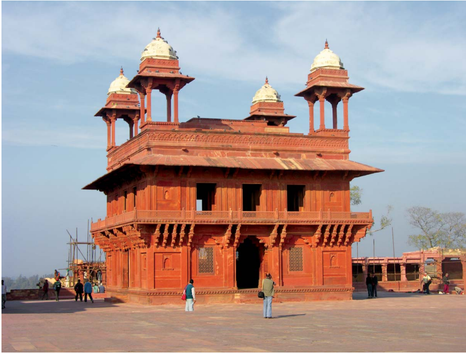
6 Diwan-i Khass (private audience hall), Fatehpur Sikri palace complex, ca. 1570 (photograph by the author)
