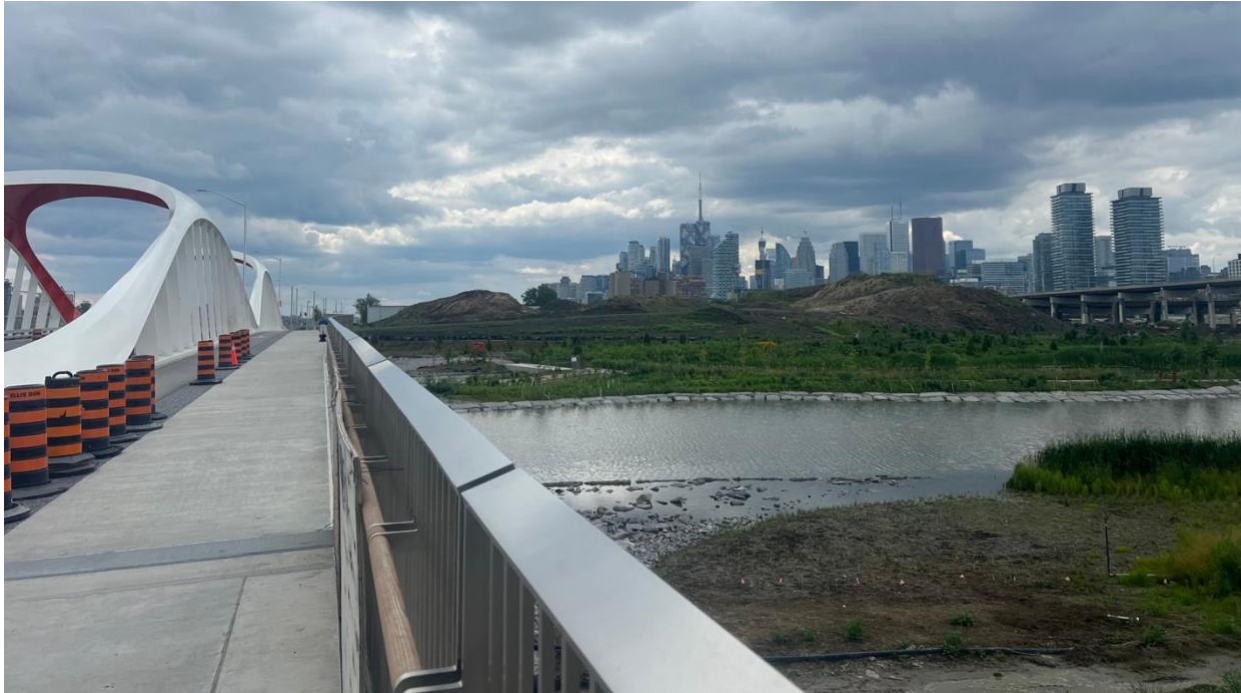
Figure 24 The Port Lands during construction, looking west toward the downtown core, July 2024. Photograph by author.
