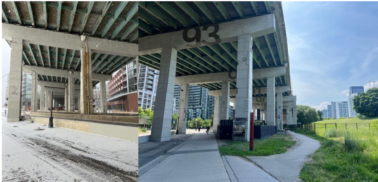
Figure 10 (left) The "cathedral-like" space under the bents of the Gardiner near Fort York Boulevard crossing in February 2024. Photograph by author.
