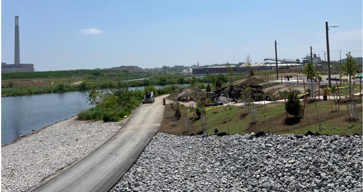
Figure 33 Construction underway for the parks on Ookwemin Minising, July 2025. Photograph by author.
