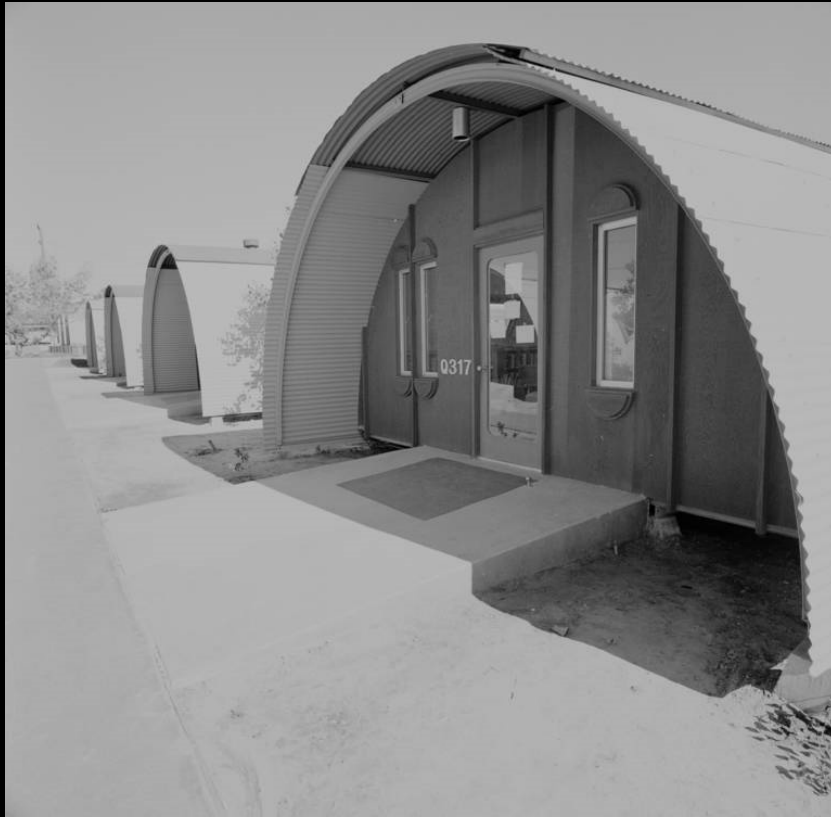
Army-era Quonset huts converted to CME studios, early 1970s
