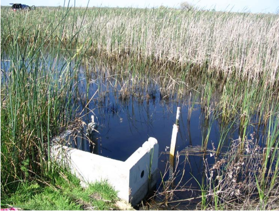
Figure 3-8: Los Banos Wildlife Management Area pond 31B outlet weir.
