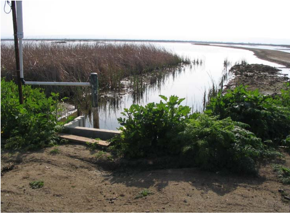
Figure 3-3: Ducky Strike North pond – drainage occurs over the outlet weir in the foreground.
