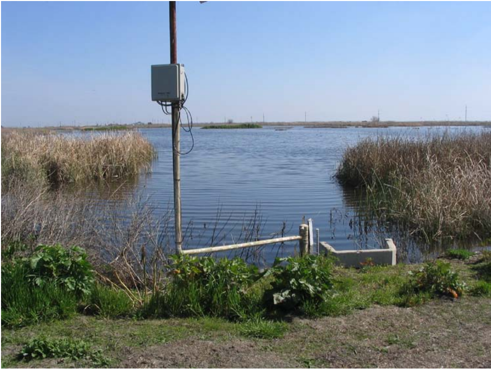
Figure 3-15: Mud Slough Wildlife Management Area pond 4B outlet weir.
