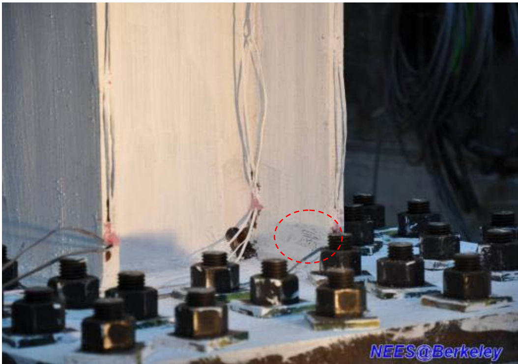
Figure 4.89 The column base at western side of TCBF-B-1 specimen
