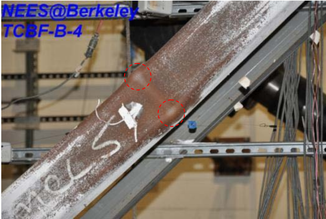
Figure 4.422 Cracks developed in the first story western side brace
