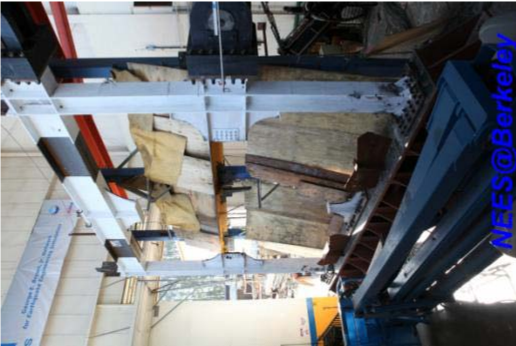
Figure 3.59 Damaged specimen after cutting off the wide flange braces
