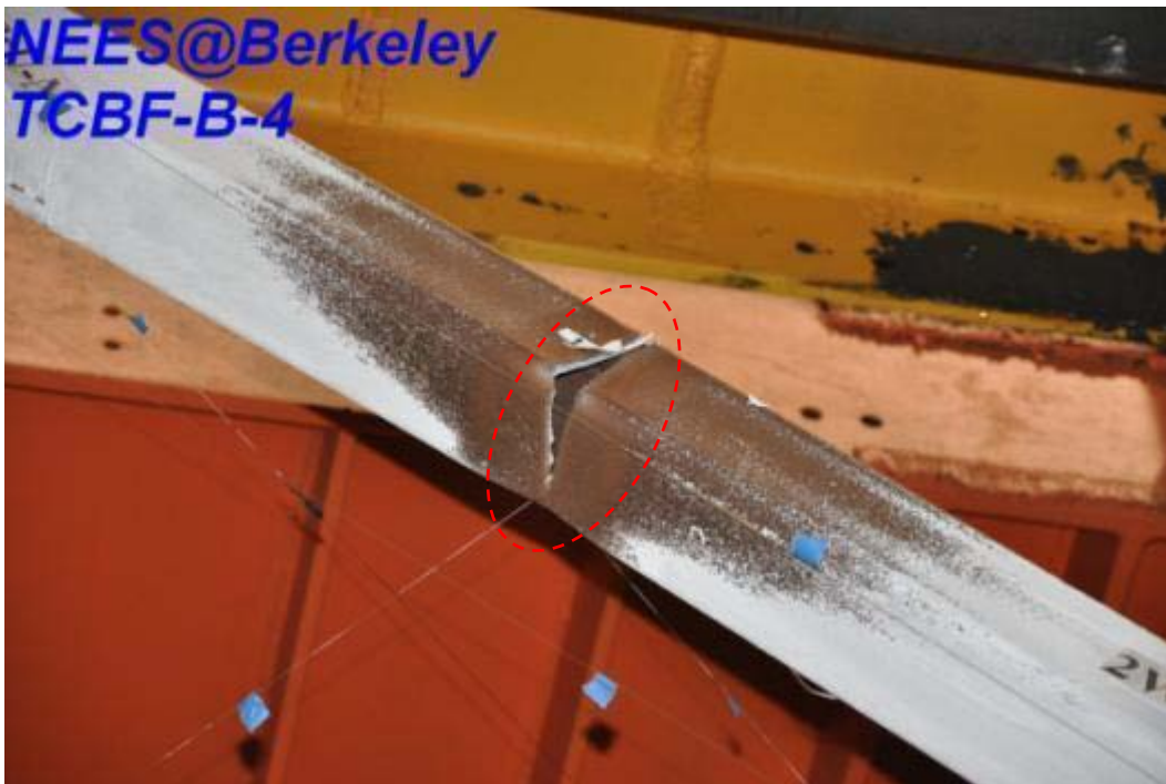
Figure 4.421 Crack propagation in the second story western side brace
