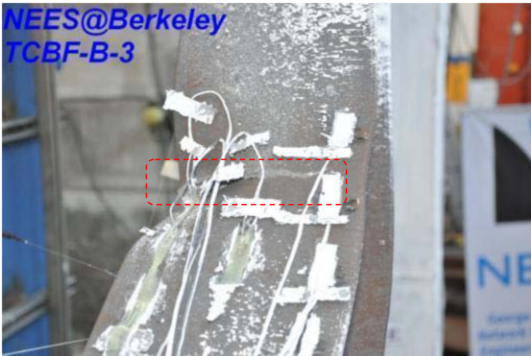
Figure 4.324 West wide flange brace partially fractured near the middle of the brace (view from east side)
