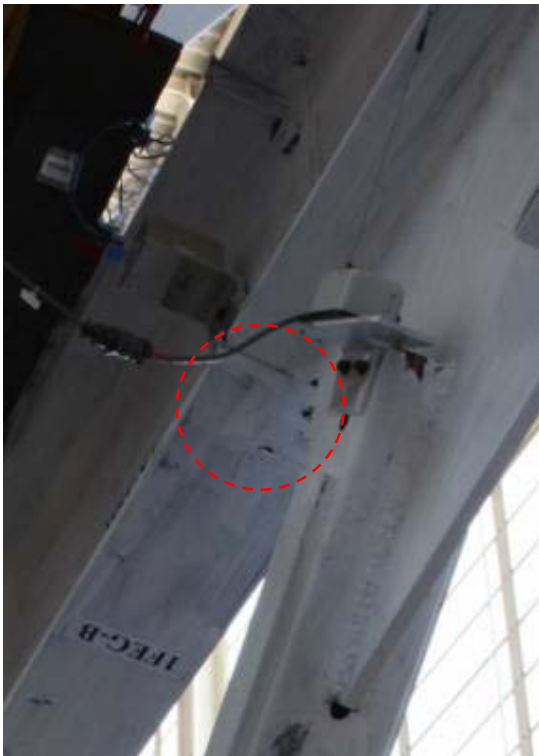
Figure 4.86 The bottom flange of east side lower beam of TCBF-B-1 specimen
