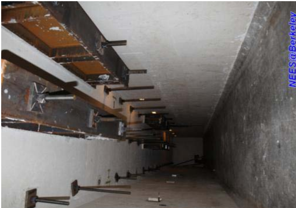
Figure 3.14 Four load transfer beams below the strong floor after pre-stressing
