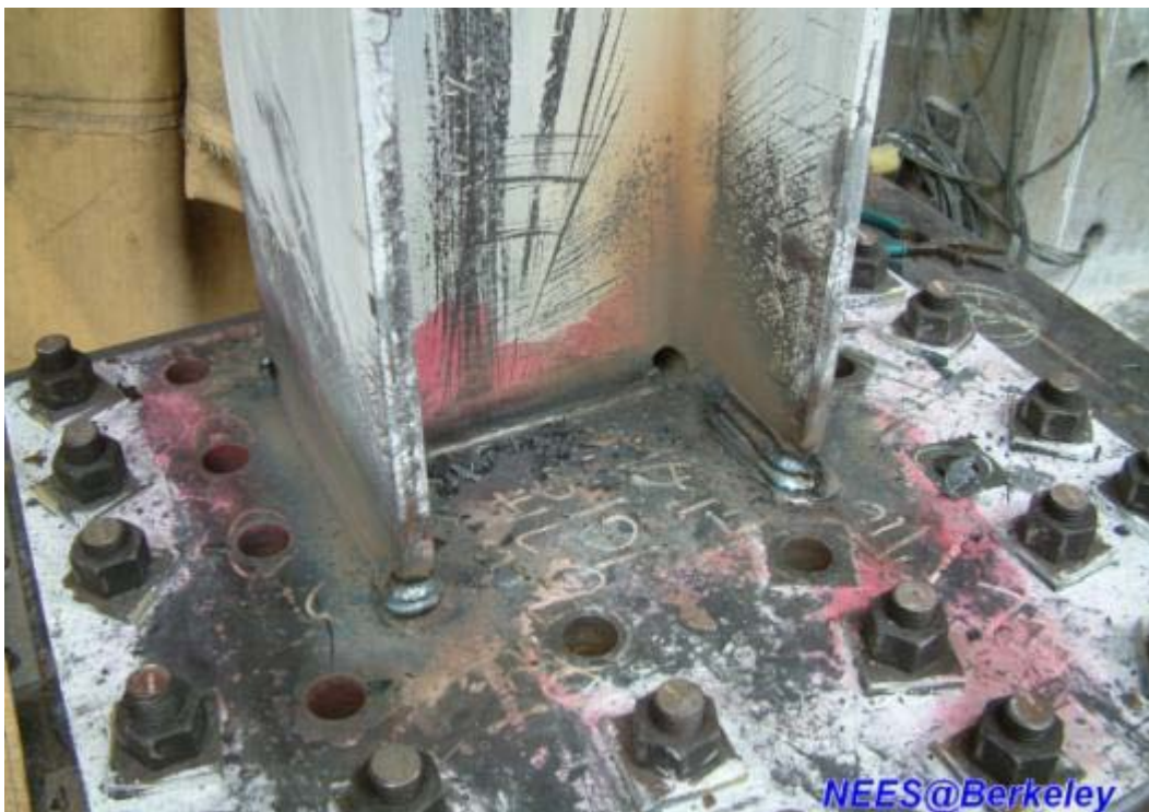
Figure 3.52 The west column base after weld repairs
