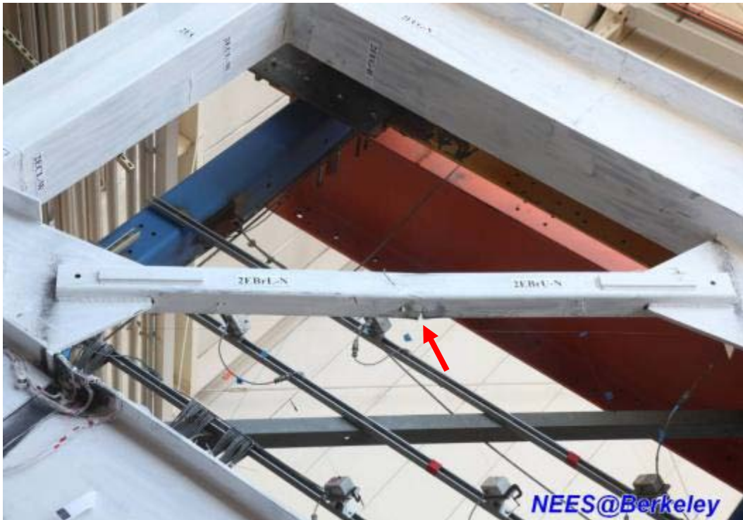
Figure 4.101 The cracks propagate in the square HSS brace at second story eastern side of TCBF-B-1 specimen
