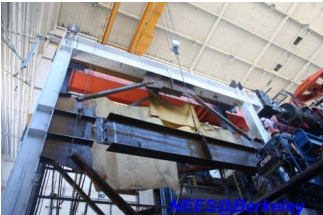
Figure 3.44 Splicing the lower beam to one-piece gusset plates in TCBF-B-2 specimen
