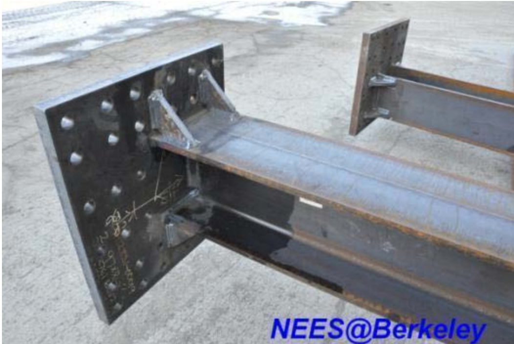
Figure 4.226 Column base connection detail of TCBF-B-3 specimen (four 7/8-in. gussets welded to the column flange and base plate)
