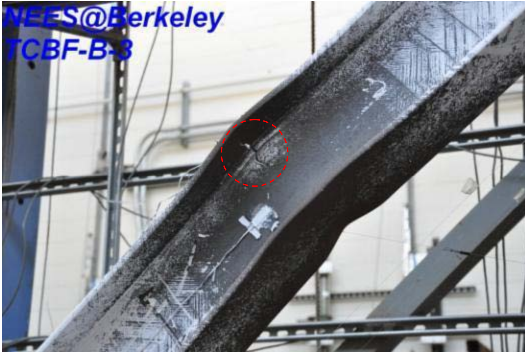
Figure 4.323 West wide flange brace partially fractured near the middle of the brace (view from north-west side)
