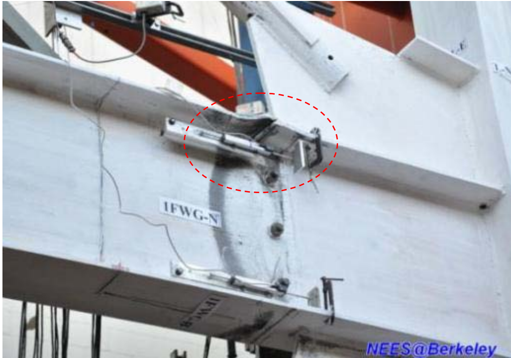
Figure 4.207 Fracture of lower beam top flange (west side of Specimen TCBF-B-2)
