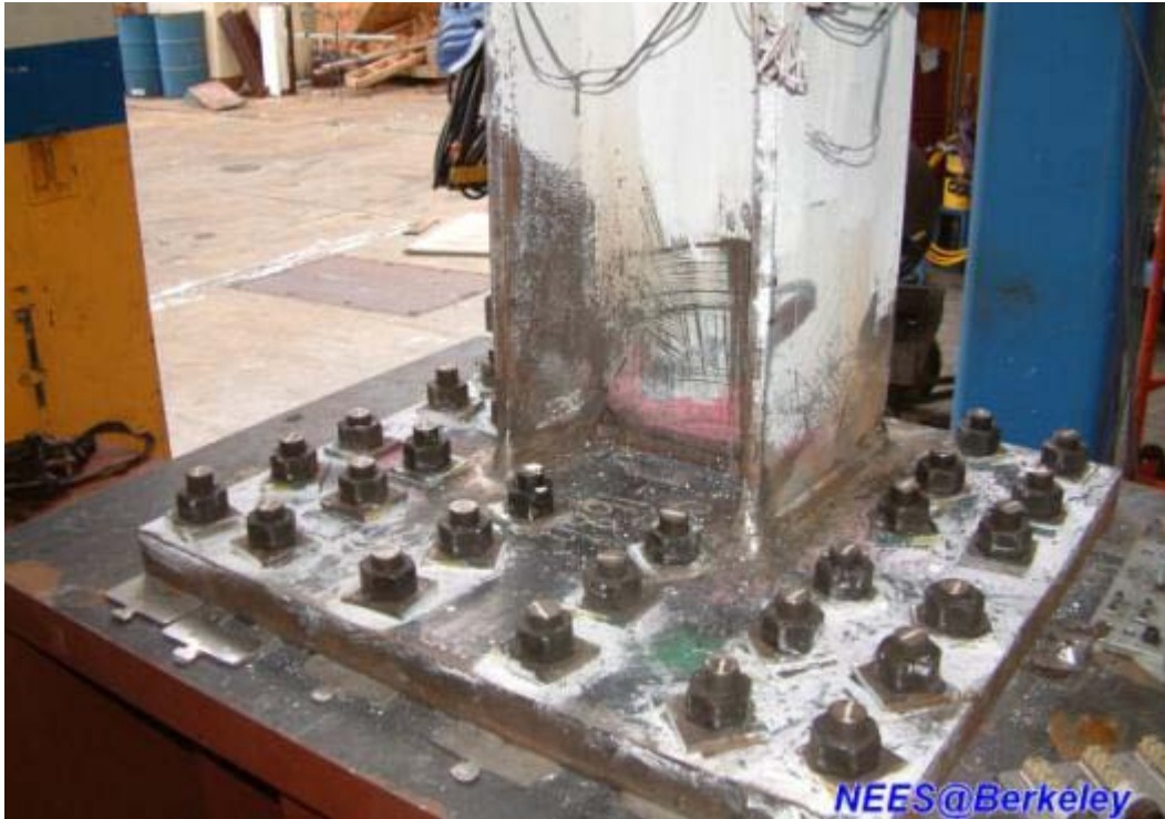
Figure 3.53 The east column base after weld repairs
