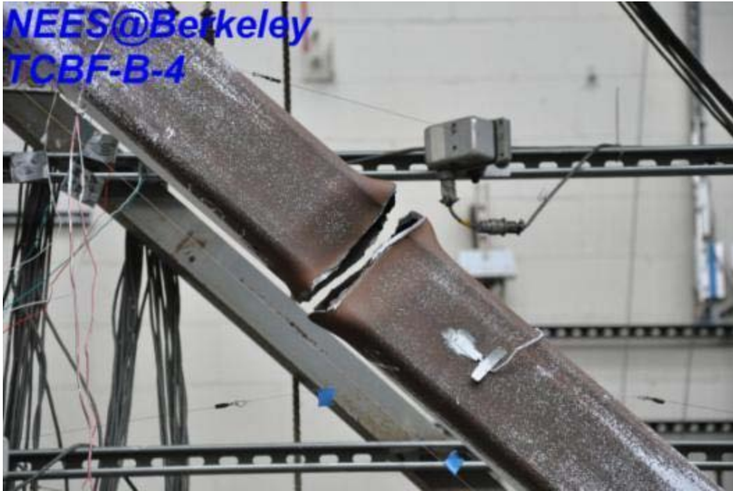
Figure 4.426 Completely fracture of the first story eastern side brace
