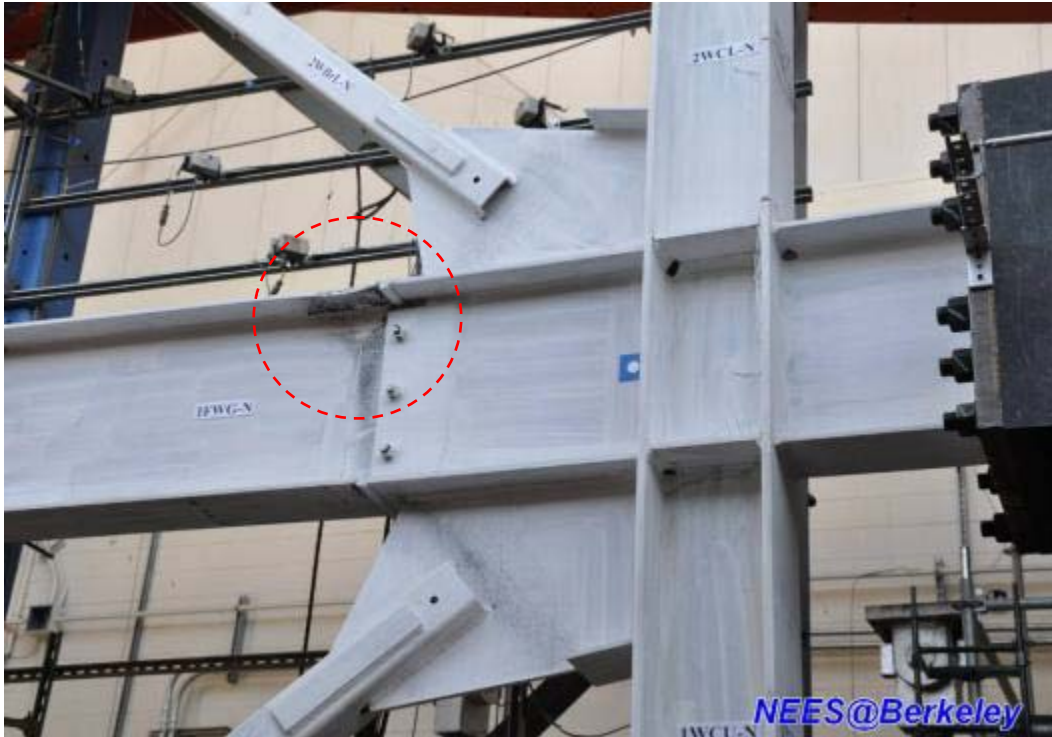
Figure 4.90 The lower beam-to-gusset plate splice at western side of TCBF-B-1 specimen
