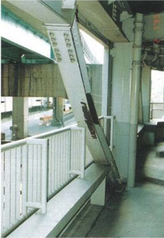
(a) Wide flange brace
