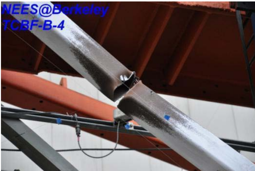
Figure 4.425 Completely fracture of the second story western side brace
