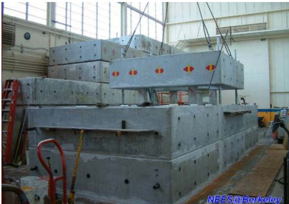
Figure 3.10 Construction of reconfigurable reaction wall before pre-stressing
