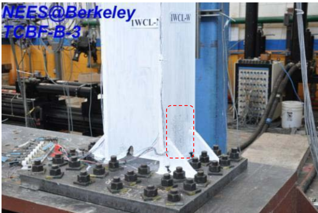
Figure 4.316 Whitewash flaking patterns shown on the column flanges near the column base plate (west column base)
