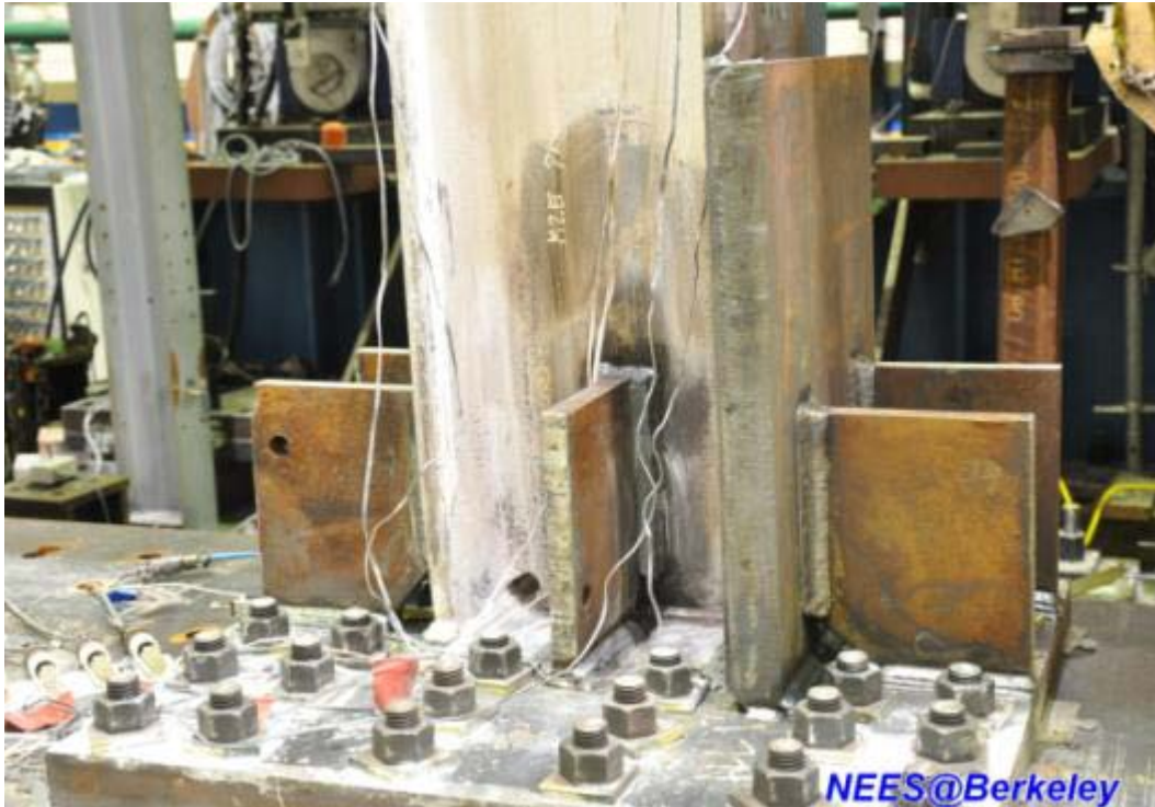
Figure 4.203 West side column base after repair (Specimen TCBF-B-2)
