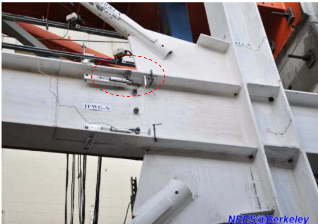
Figure 4.198 Local buckling of lower beam top flange at west side (Specimen TCBF-B-2)
