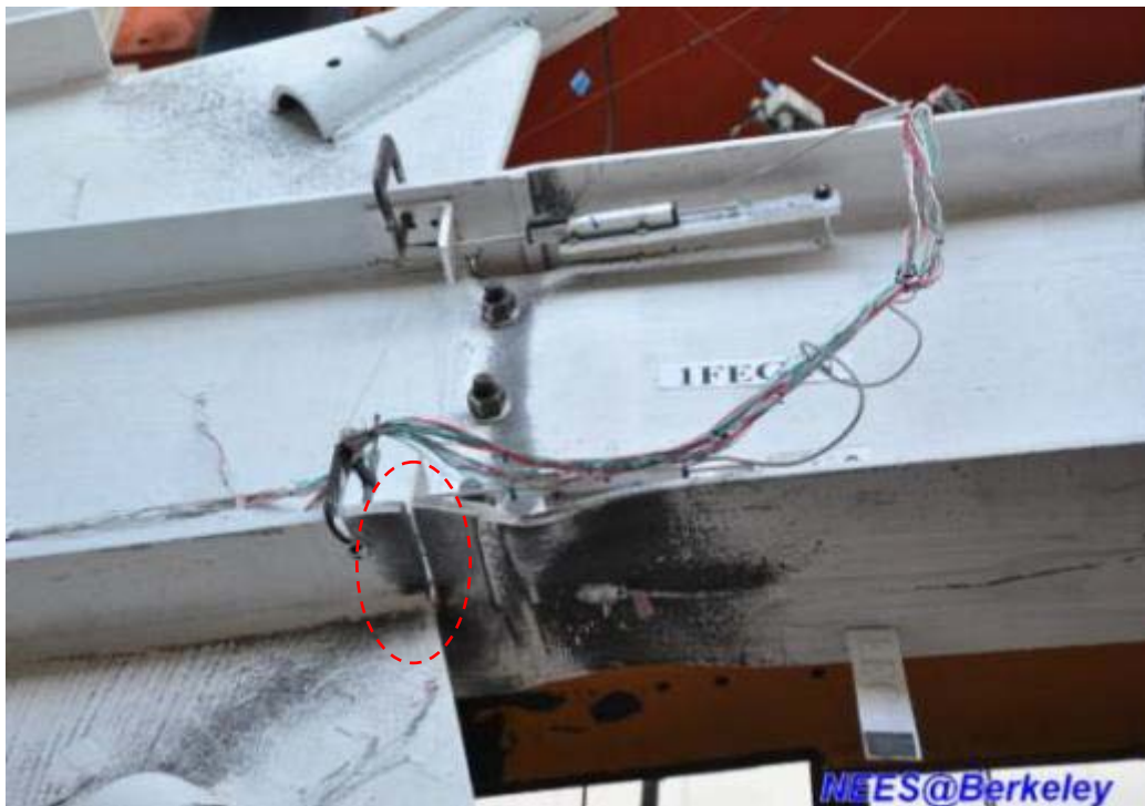
Figure 4.208 Partial fracture of lower beam bottom flange finger plate (east side of Specimen TCBF-B-2)
