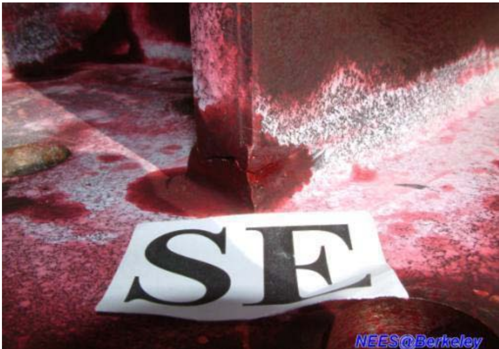
Figure 3.50 Crack detecting spray applied in the CJP weld at east column base (south-east corner)
