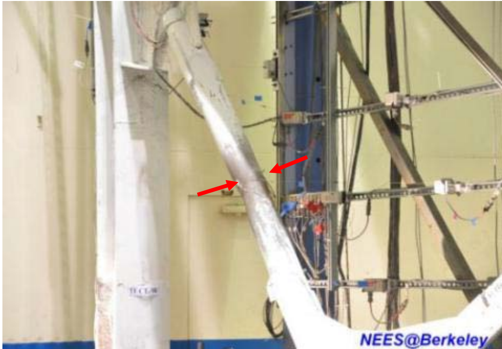
Figure 4.223 Necking of the east side round HSS brace in the first story before fracture
