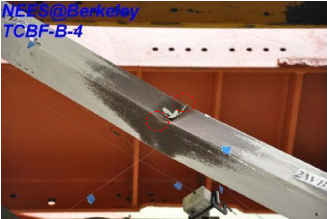
Figure 4.420 Cracks in the second story western side brace
