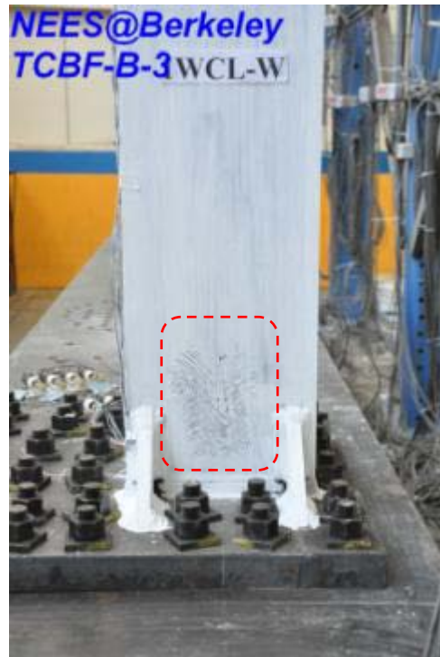
(b) West column base
