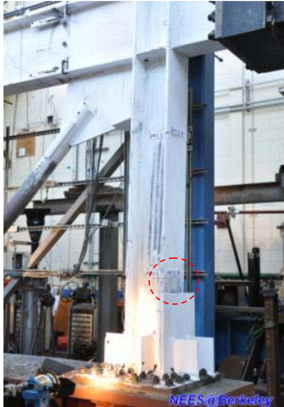
Figure 4.205 Yielding in the column flange near 2-in.-thick cover plate (Specimen TCBF-B-2)
