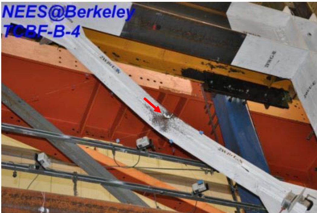
Figure 4.415 Local buckling of western side brace in the second story
