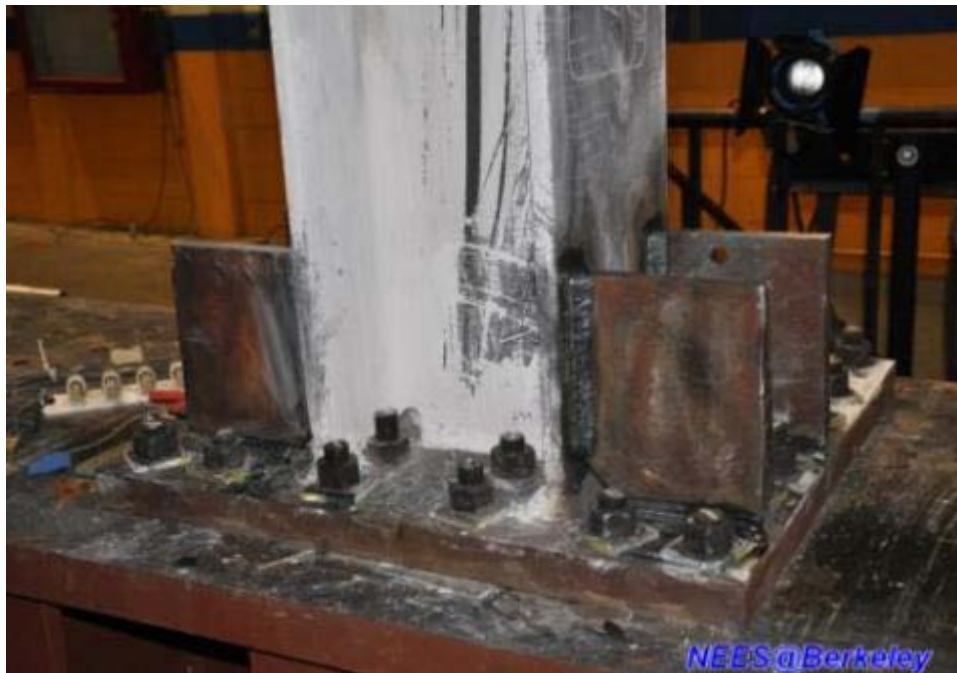
Figure 4.204 East side column base after repair (Specimen TCBF-B-2)
