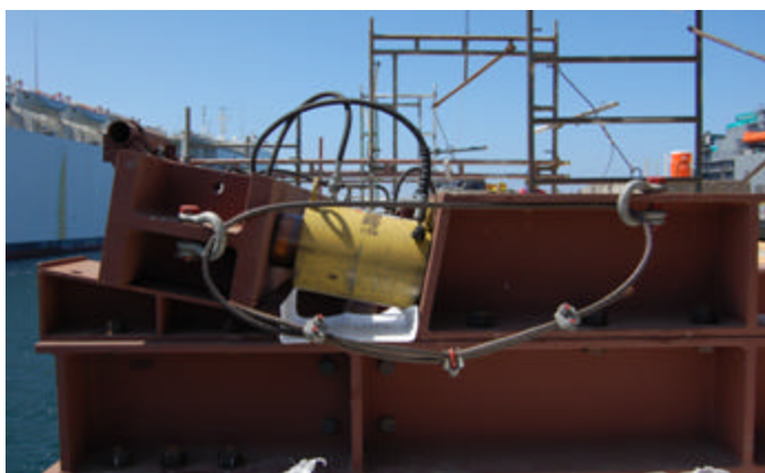
(c) Cross-Beam and Hydraulic Jacks at 11°
