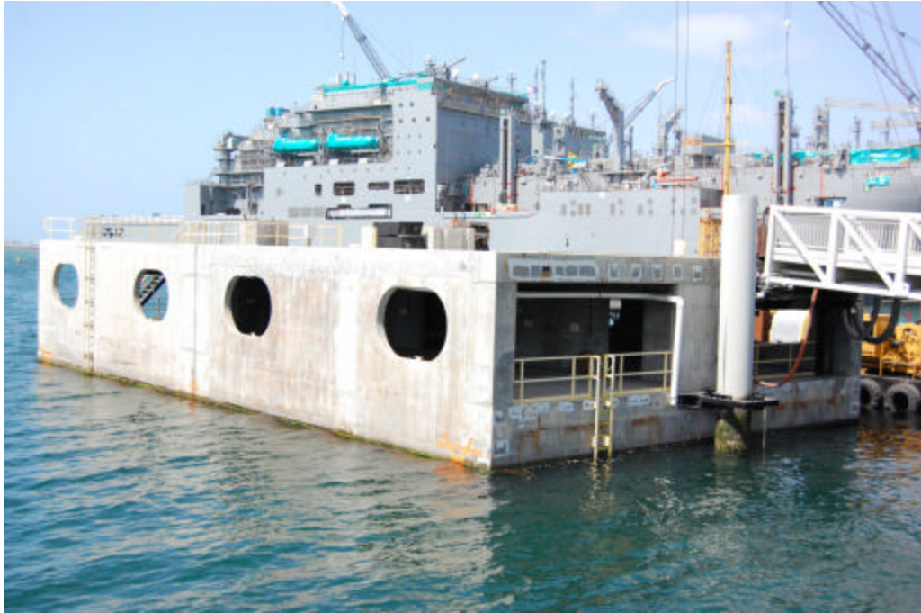
Figure 1.1 - Photograph of MHP - Southeast End
