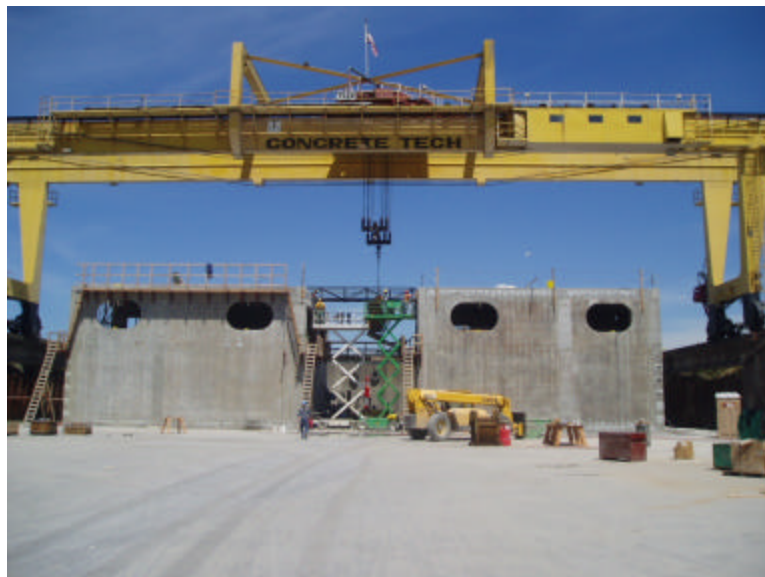
Figure 1.2 - MHP Test-Bed Structure in Dry Dock
