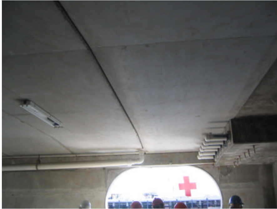
Figure 2.4 - Bottom View of Prestressed Precast Planks
