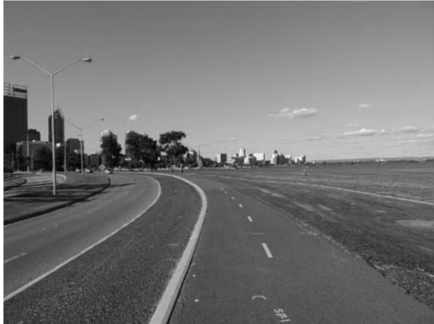
Figure 23: Physical separation of pedestrian and cycle modes via concrete curbing.
