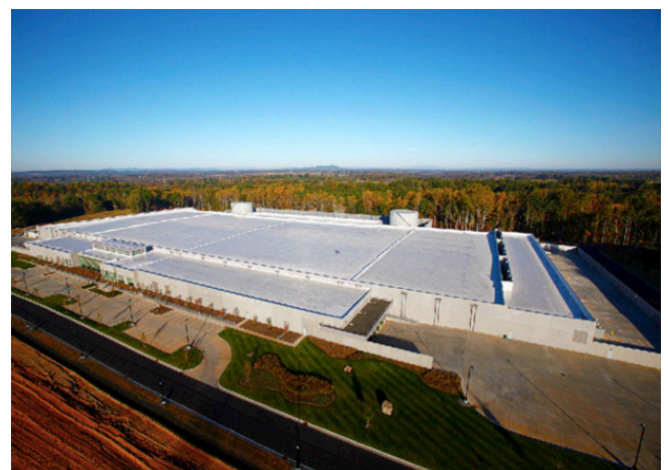
Fig. 3 Data Centers are becoming integral parts of a new semiotic infrastructure.
