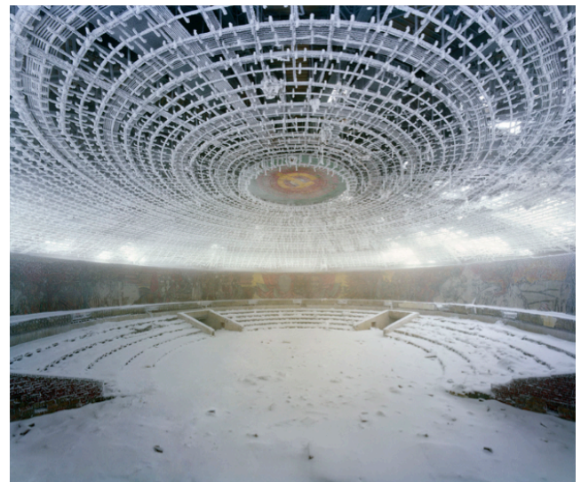
Fig.1. When maintenance and repair stop and meanings collapse. Abandoned headquarters of the Bulgarian communist party. Photo by Thomas Jorion .
