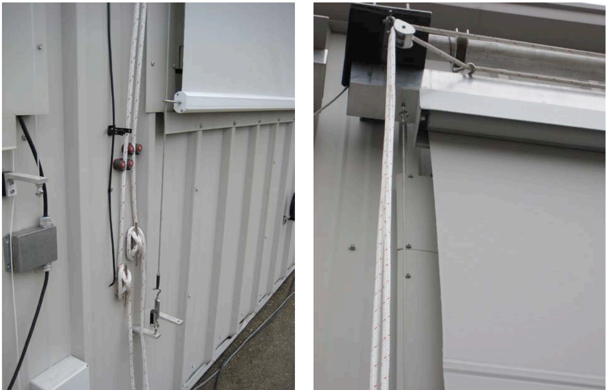
Figure 30: Views of lower hem bar (left) and header (right) mounted on the hoist system.
