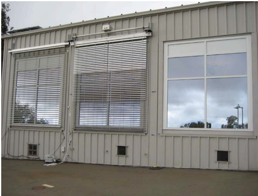
Figure 6: Exterior view of the LBNL Windows Testbed Facility with the VB-E1n and VB-E3opt systems installed on the left and middle test chamber windows, respectively. The reference case with an interior Venetian blind (reference-VB) is on the right-most chamber window.
