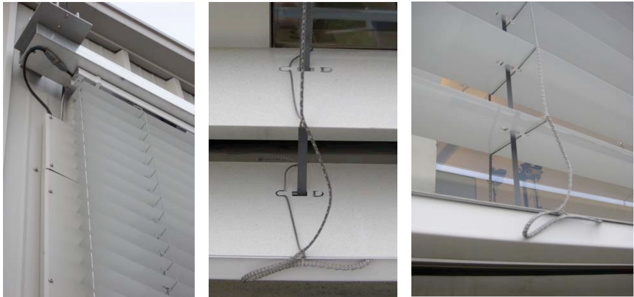
Figure 29: Views of header (below hoist beam), top of slat, and underside of slats.
