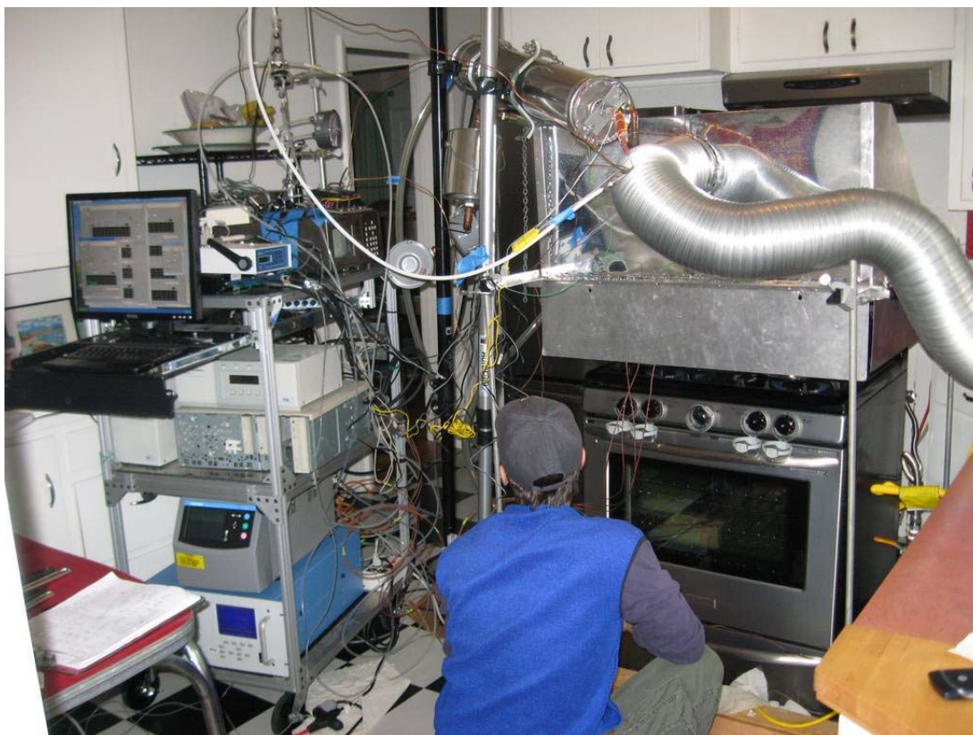
Figure 7. Collection hood installed over island cooktop
