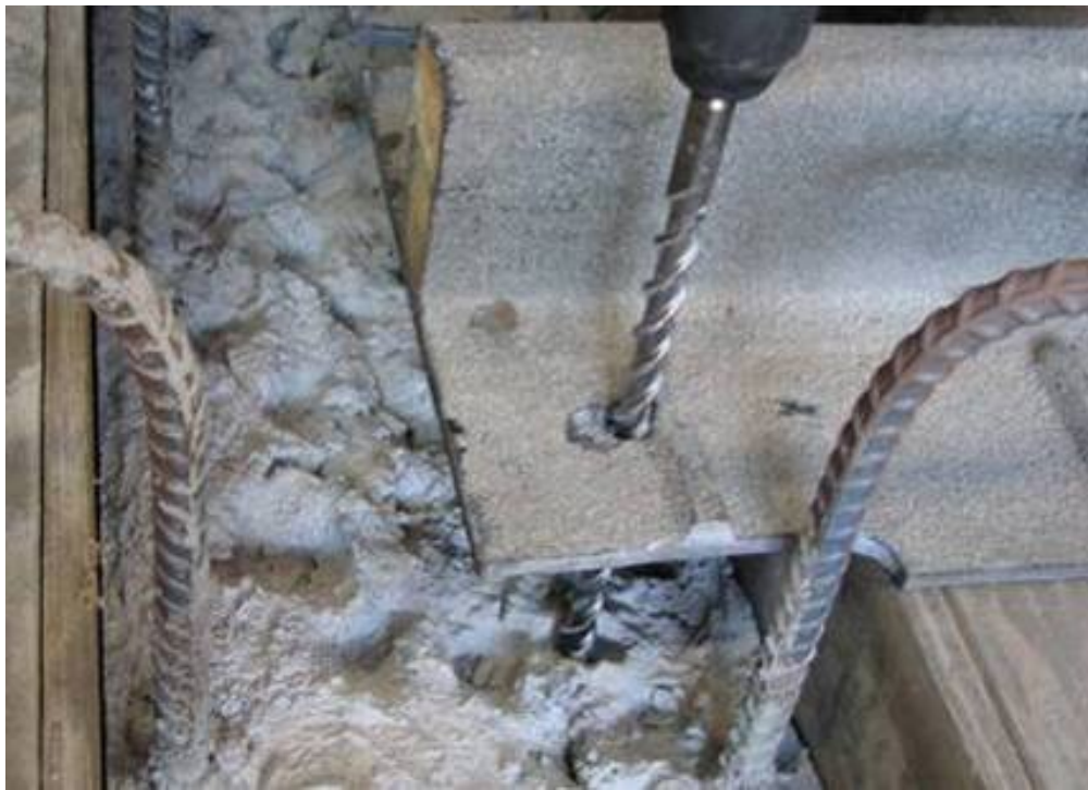
Figure 5.5 Drilling of stem concrete using FRP panels for alignment of holes
