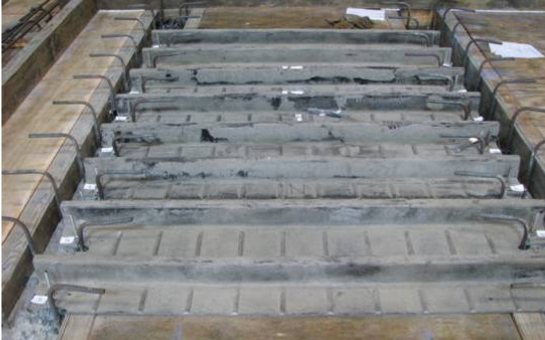
Figure 5.7 Composite side deck after FRP panel installation
