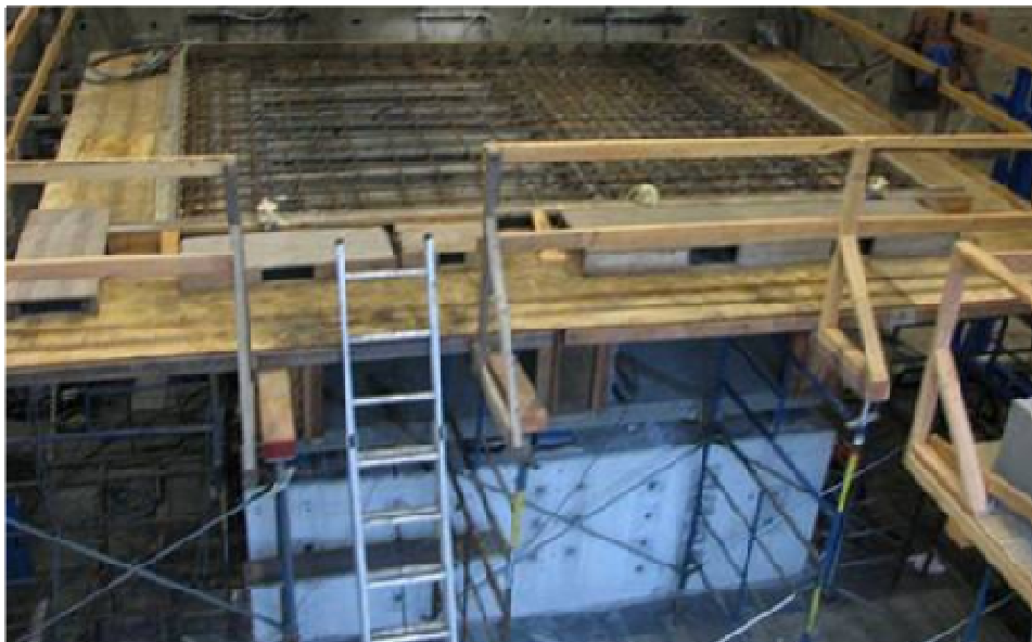
Figure 5.2 Construction of test specimen formwork for 2nd pour
