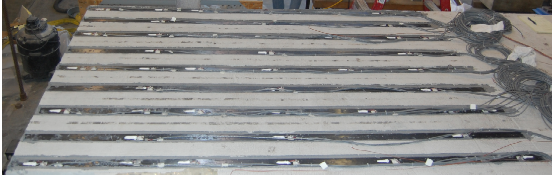
Figure 6.32 CFRP strips installed
