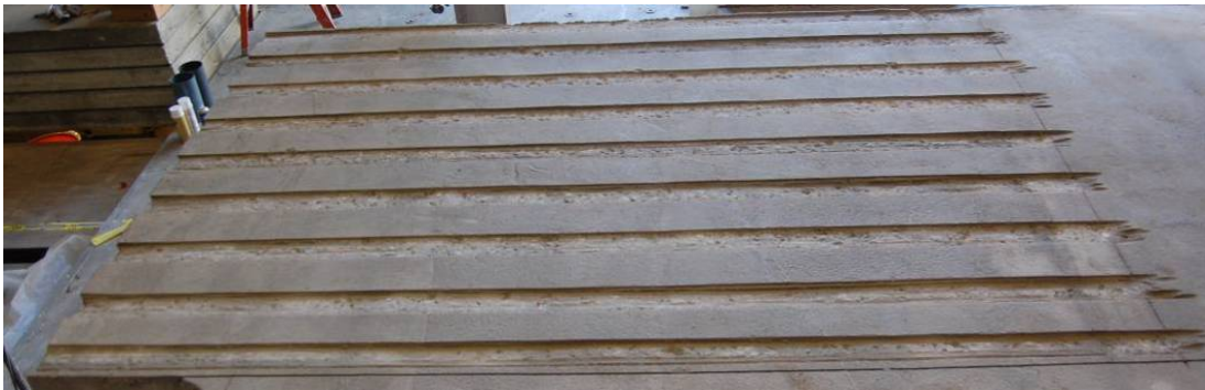
Figure 6.30 Grooves cut in deck for NSM strengthening
