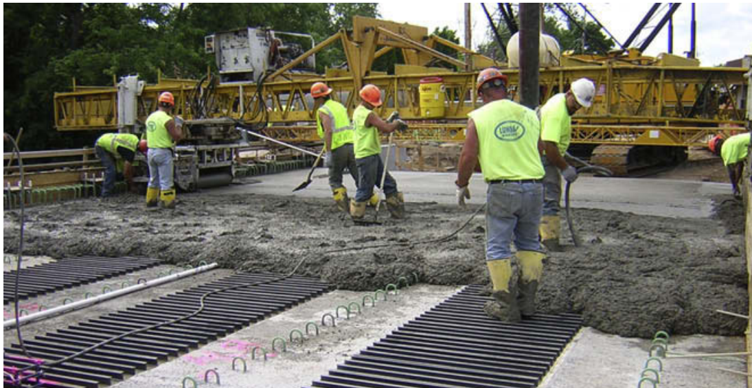
Figure 2.6 Use of commercially available FRP plank as SIP formwork and secondary reinforcement in reinforcement-free deck [66]
