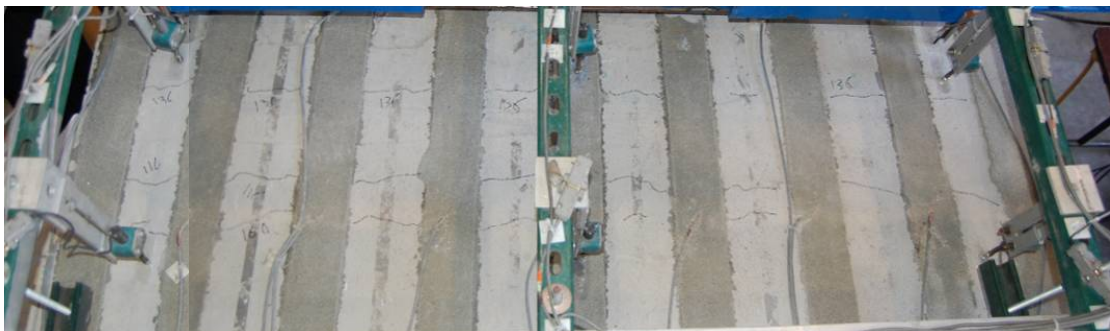
Figure 6.43 Cracking of deck slab at ultimate capacity- top view of deck
