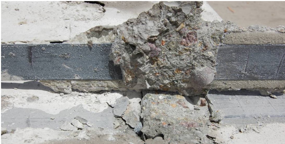
Figure 6.58 Detail of failure surface of FRP strip
