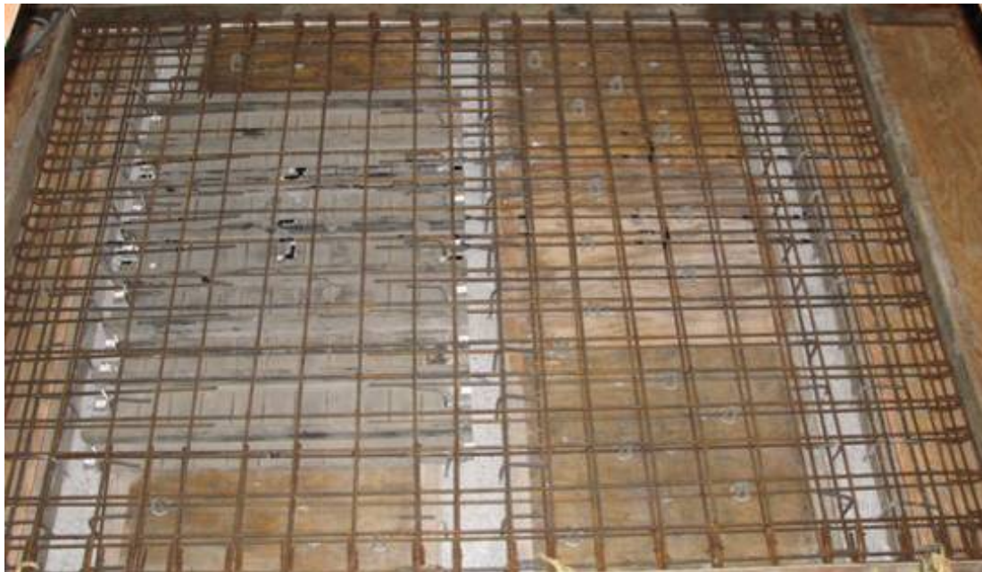
Figure 5.8 Reinforcement system in deck, as built
