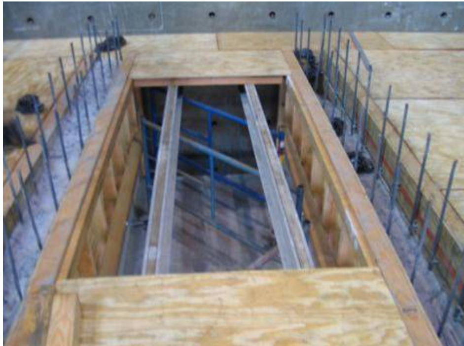
(a) Composite side deck prior to FRP panel installation
