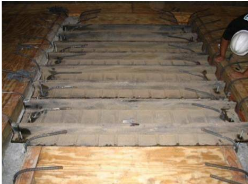
(b) Composite side deck after FRP panel installation
