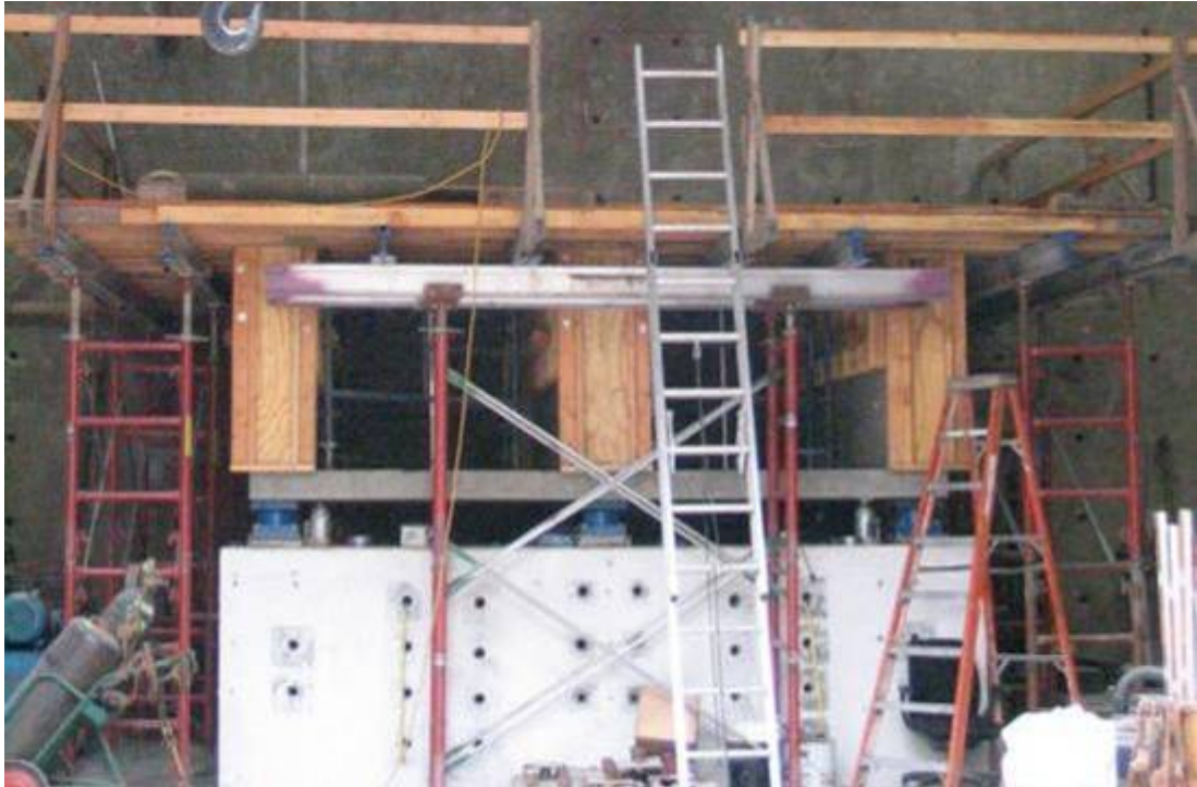
Figure 3.9 Construction of test specimen formwork for 2nd pour
