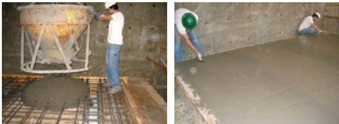
Figure 3.10 Pouring of deck concrete and finishing of deck surface
