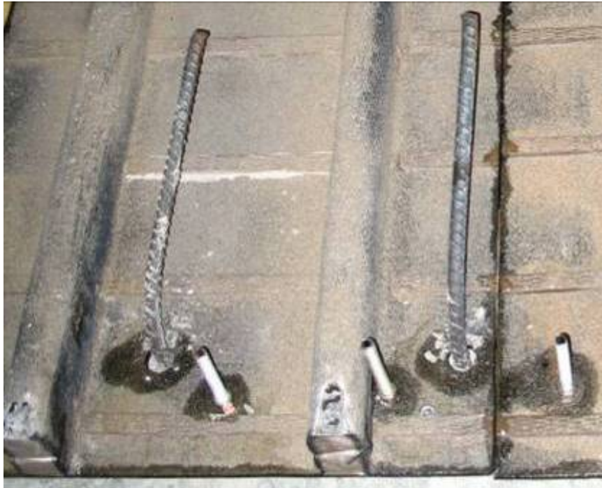
(a) End condition detail from Test Specimen #1.
