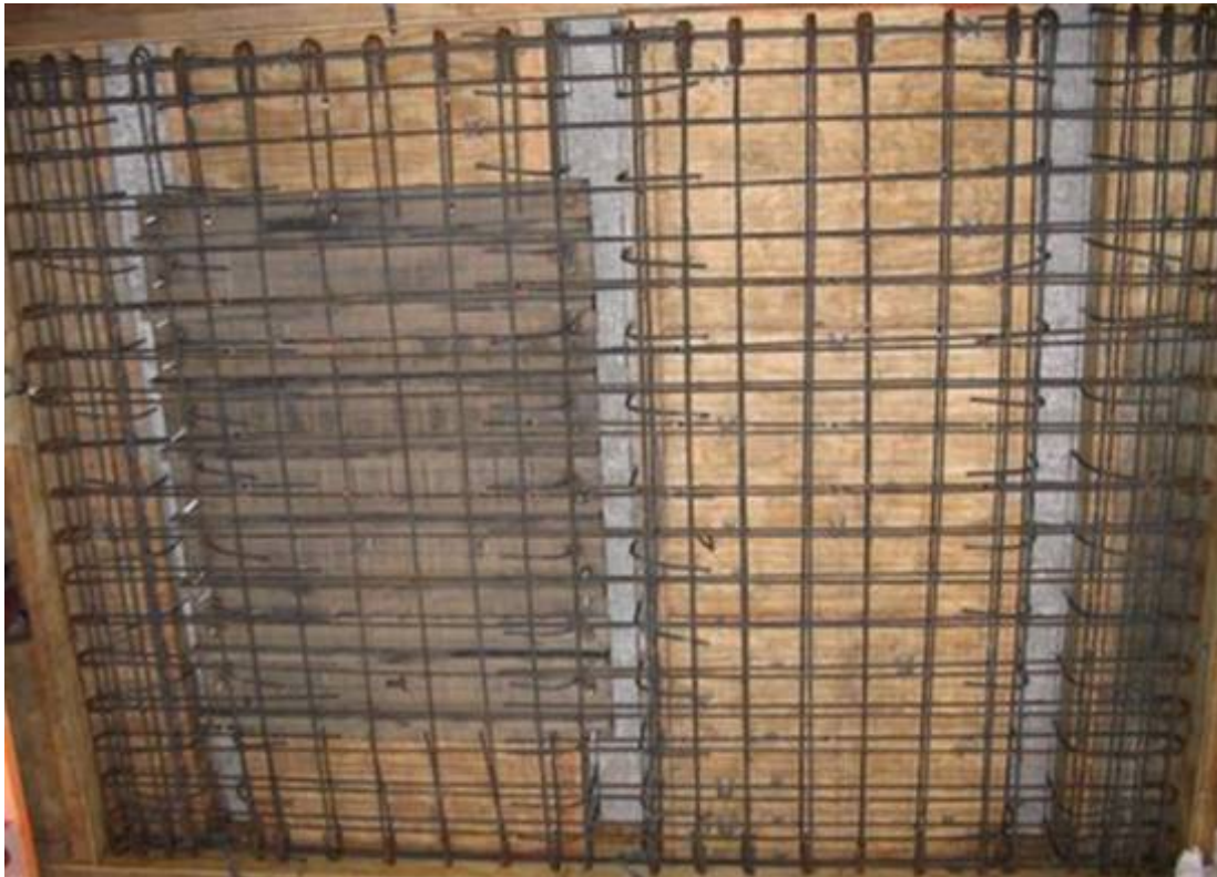
Figure 3.15 Plane view looking down on reinforcement system in deck, as built
