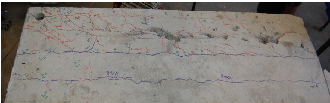
Figure 6.19 Cracks observed on top of slab tested to ultimate capacity
