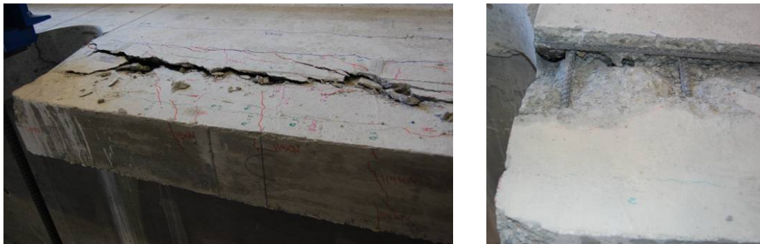
(a) Edge of deck prior to loose concrete removal
