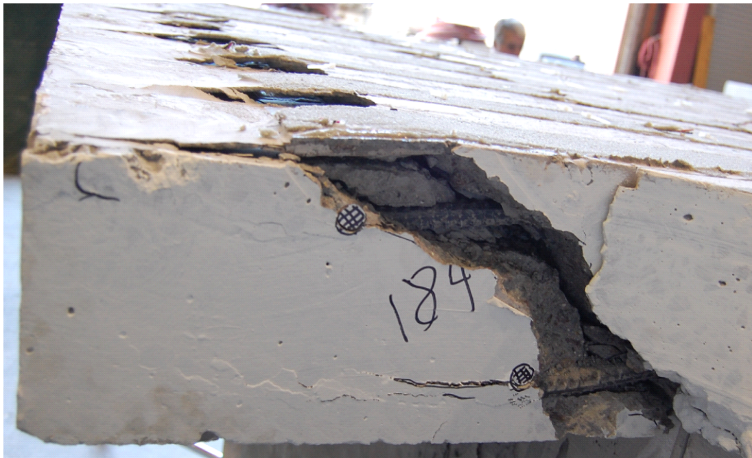
Figure 6.44 Side view of tested FRP rehabilitated specimen after removal of loose concrete
