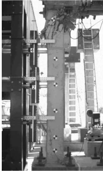
Figure 3.20: Advanced Damage Pattern (Test 3, 69.3 ms)
