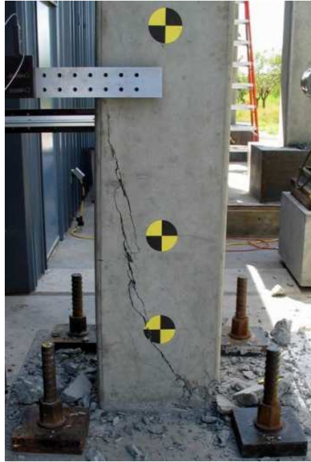
Figure 3.24: Damage Pattern Bottom Right (Test 3)
