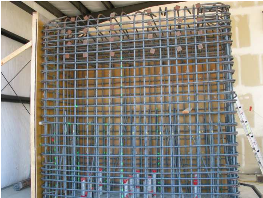
Figure 2.24: Fixed Wall Reinforcement (15 Oct, 2004)
