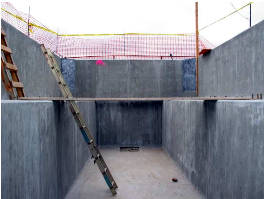
Figure 2.16: Finished Foundation From Inside (3 Oct, 2003)
