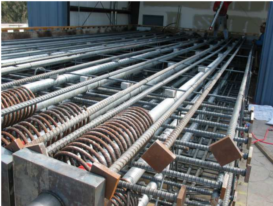
Figure 2.20: Main Slab Reinforcement (9 Sep, 2004)
