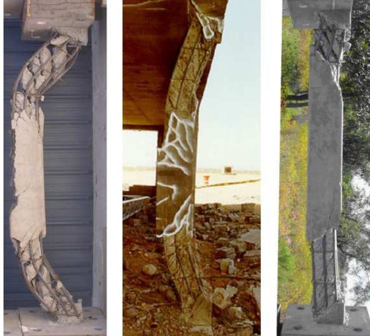
Figure 4.2: As-Built Columns: Test 2 (Left), DB6 (Center), and Test 7 (Right)
