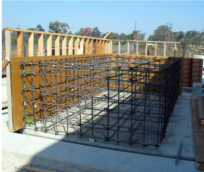
Figure 2.25: Moveable Block Reinforcement (15 Oct, 2004)
