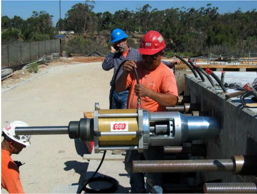
Figure 2.21: Main Slab Post-Tensioning (27 Sep, 2004)
