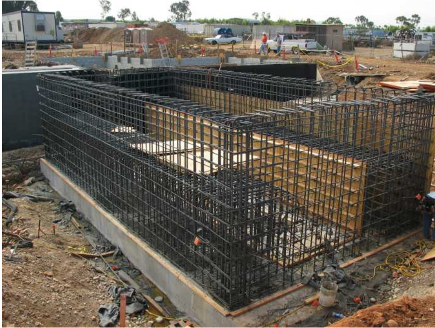
Figure 2.13: Foundation Rebar Cage (12 Aug, 2003)
