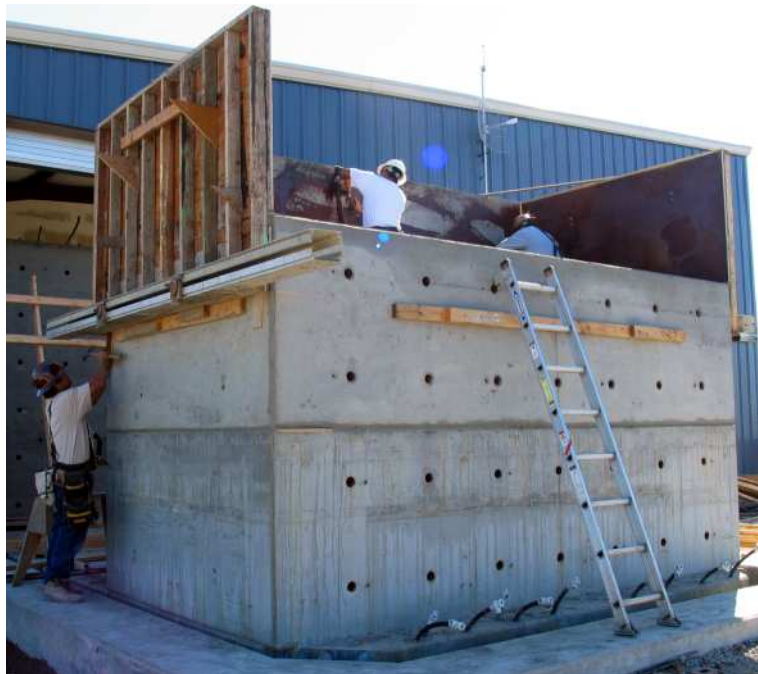
Figure 2.26: Two Blocks of Moveable Wall (2 Nov, 2004)
