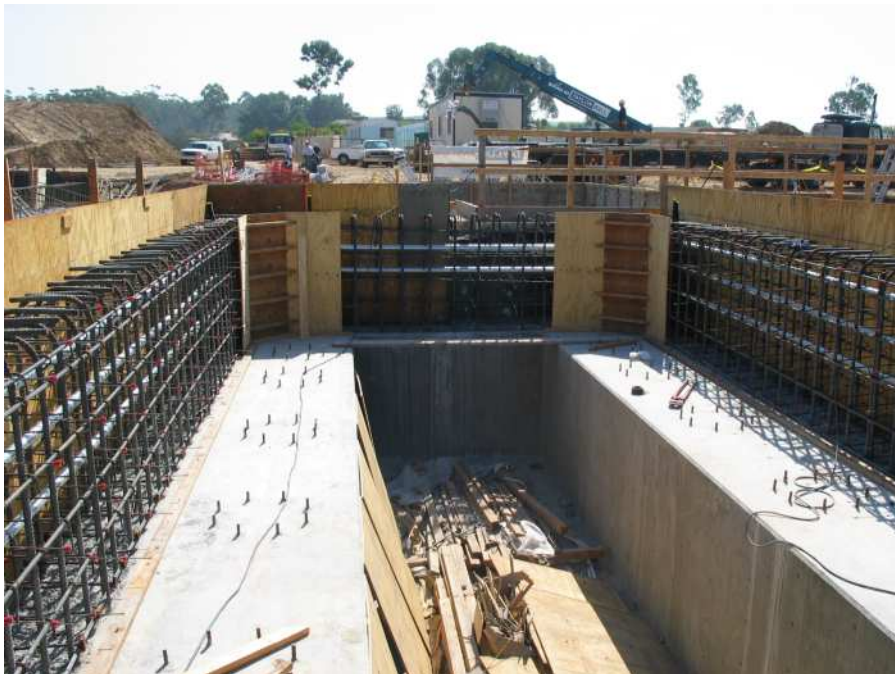
Figure 2.14: Isolator Pedestals and Upper Foundation Rebar (29 Aug, 2003)
