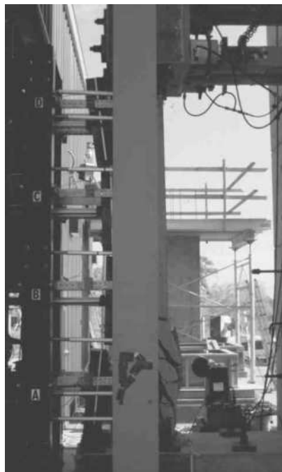
Figure 3.61: Damage Progressing (Test 8, 36.9 ms)
