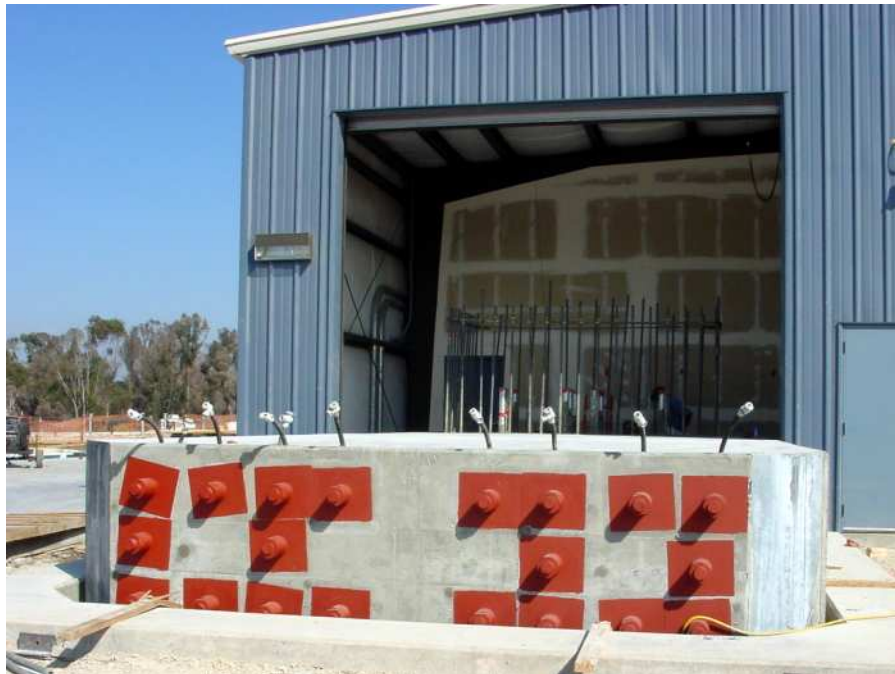
Figure 2.22: Main Slab Lowering (courtesy of L. Berman, 6 Oct, 2004)
