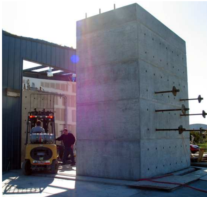
Figure 2.28: Finished Moveable Wall (8 Feb, 2005)
