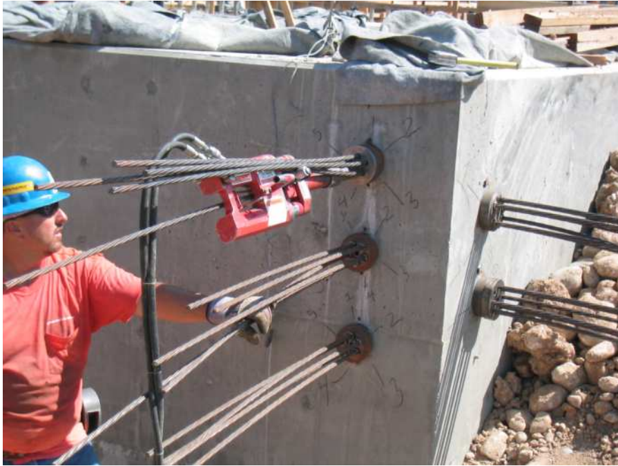
Figure 2.15: Foundation Post-Tensioning (courtesy of C.S. Lee, 16 Sep, 2003)
