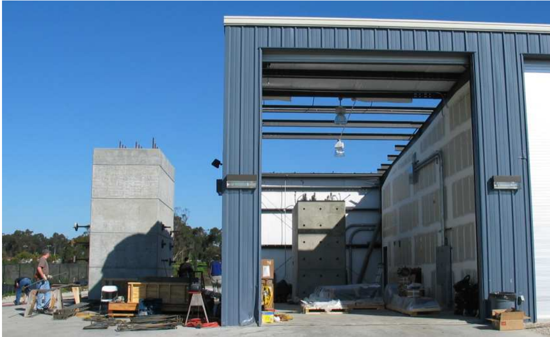
Figure 2.27: Completed Testing Superstructure (8 Feb, 2005)
