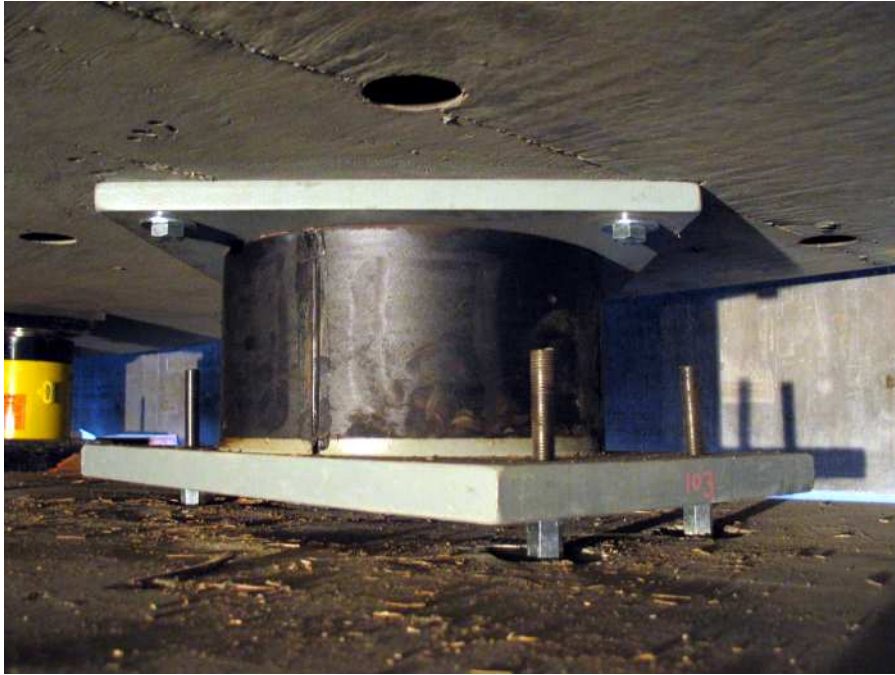
Figure 2.23: Isolators and Jack (15 Oct, 2004)
