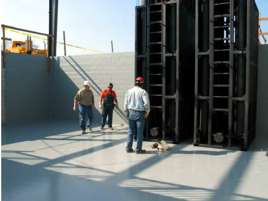
Figure 2.17: Installation of Accumulator Banks (5 Nov, 2003)
