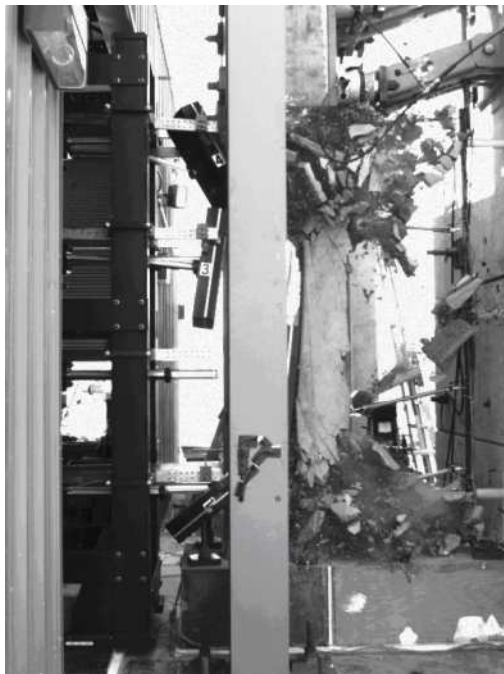
Figure 3.11: Column Failure Continues (Test 2, 112 ms)
