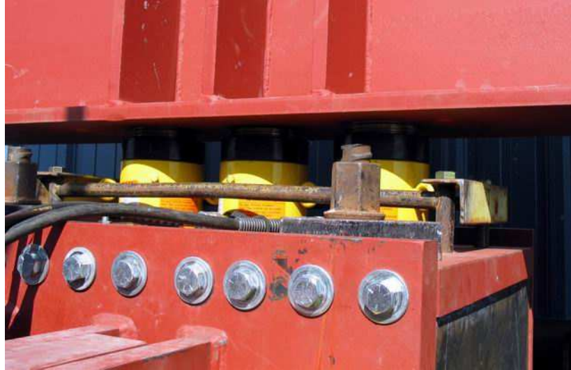
Figure 3.2: Hydraulic Jacks for Vertical Load
